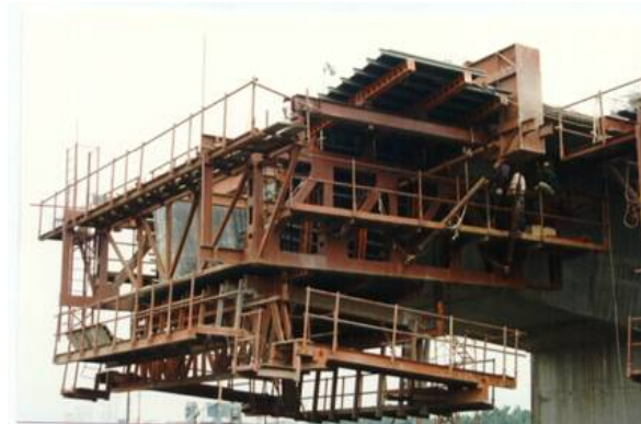
Ilan Bridge, Taiwan (Max. segment weight 120t, FT steel weight 55t)
