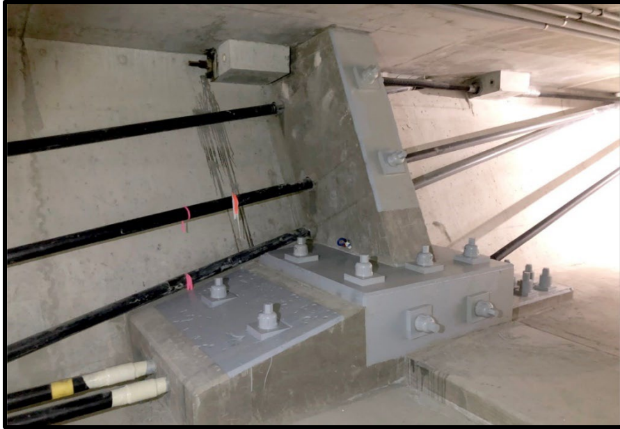
New anchor/deviator designed to anchor and deviate new draped tendons
