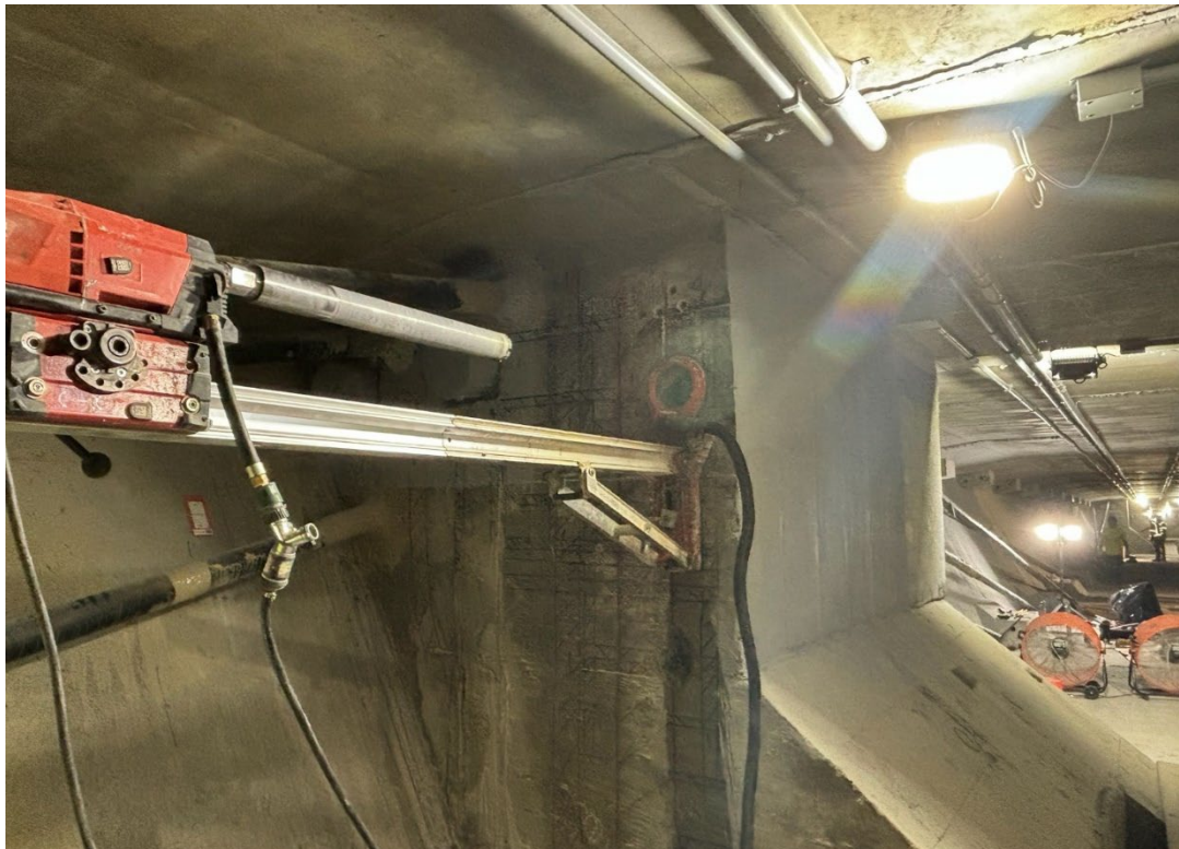
Diaphragm coring for new tendons. Note CFRP sheet used on the right face of the diaphragm to resist anchorage general zone bursting forces. (Photo from Structural Technologies)
