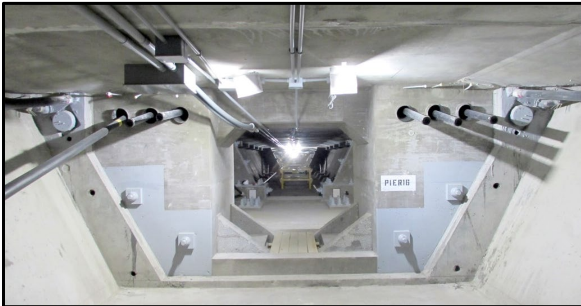
New pier segment deviator designed to deviate up to six future tendons
