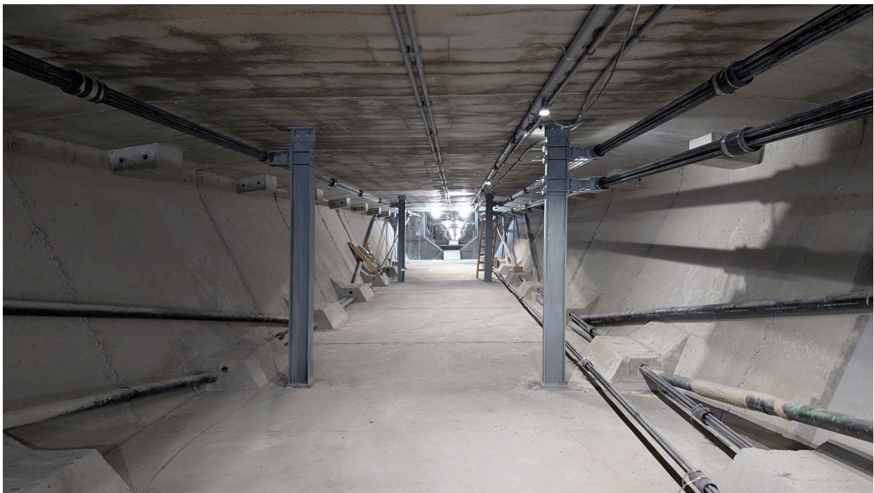
Anti-Vibration Posts for new 12-strand tendons. The upper connection of the post is designed to move in order to avoid transferring traffic load.
