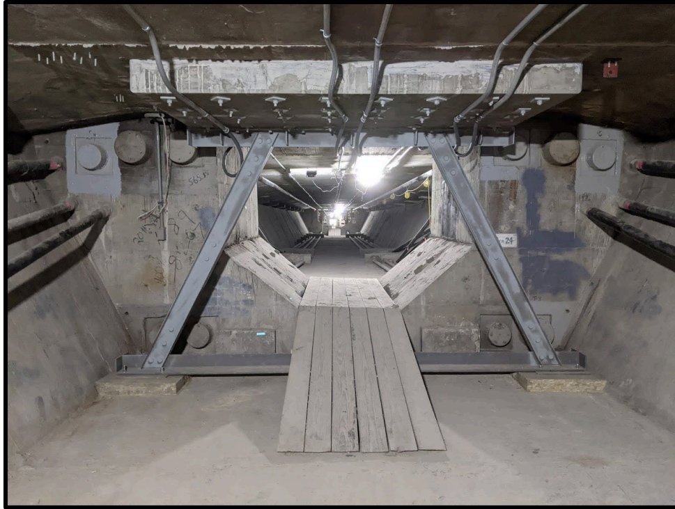
Frame and precast drop slab used to stabilize a damaged segment joint
