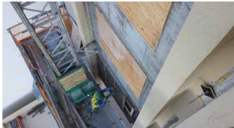
Fig. 10—Exterior shear walls.
