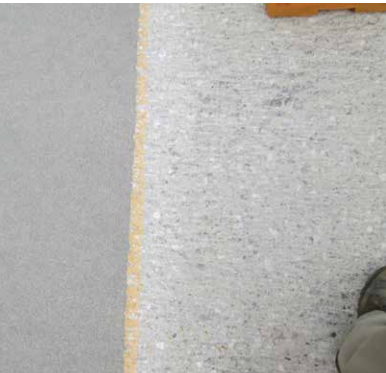
Fig. 14—Before and after concrete resurfacer.
