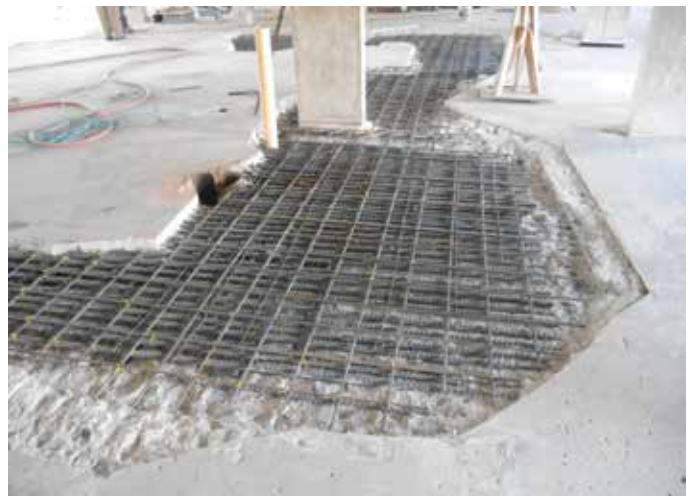
Fig. 4—Level 4 crack repair.
