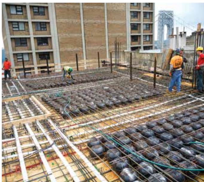
Fig. 4—PT and void formers.
