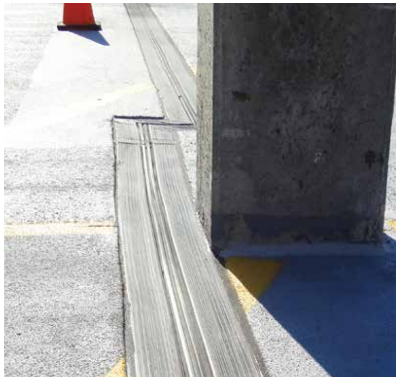
Fig. 16—Column Line 9 new expansion joint and coating.
