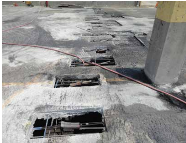
Fig. 12—Top deck PT repairs.
