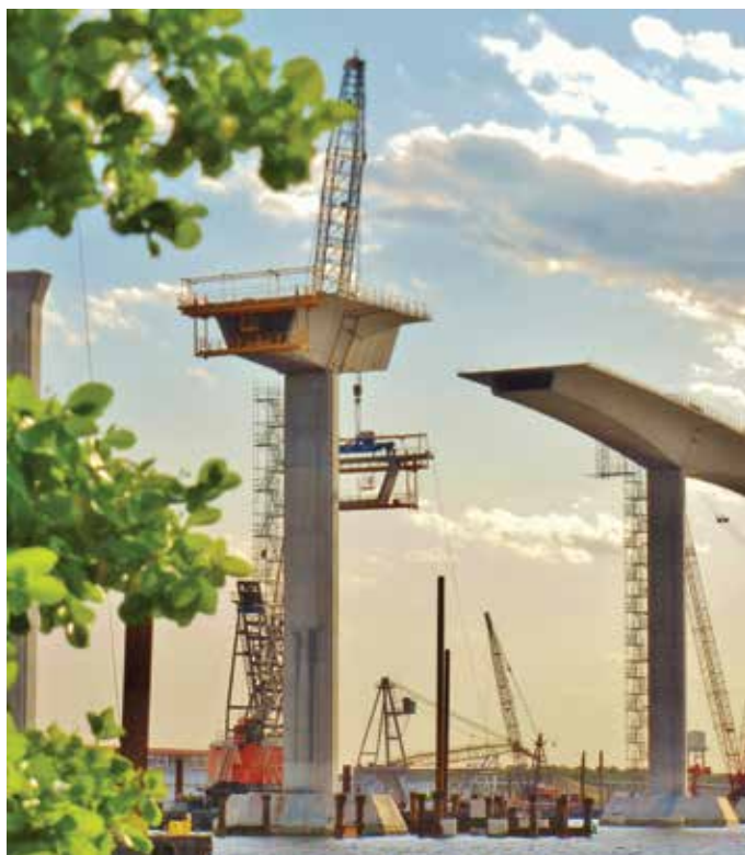
Fig. 3—Balanced cantilever construction.
