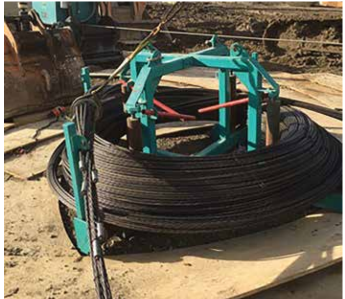
Fig. 8—Prefabricated tendons shipped to site ready for installation.
