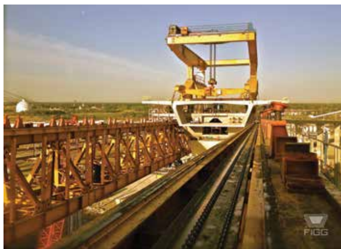
Fig. 5—Post-tensioned segmental concrete construction.
