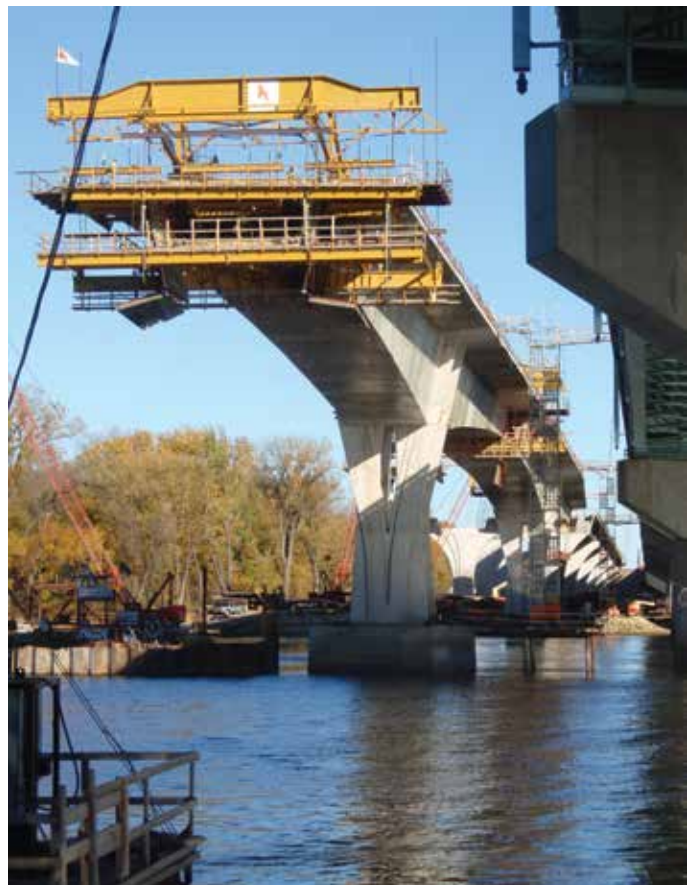
Fig. 2—Form travelers in balanced cantilever.
