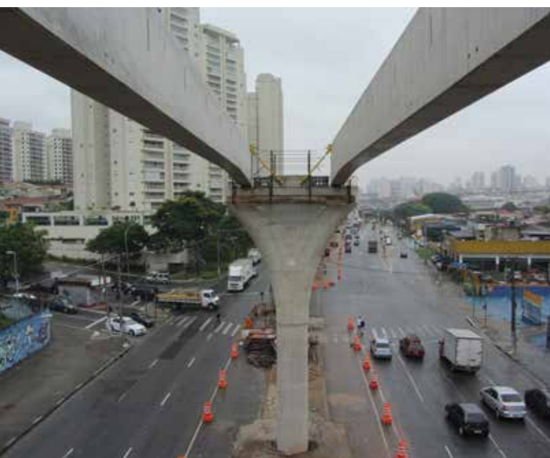
Fig. 10—PT beams during construction.
