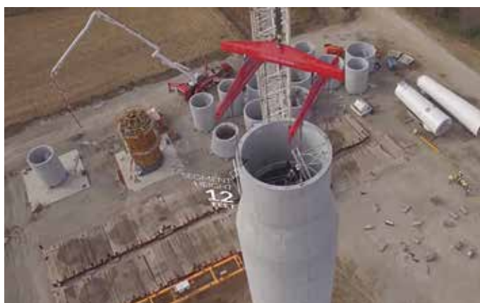
Fig. 6—Stepped concrete tower design.
