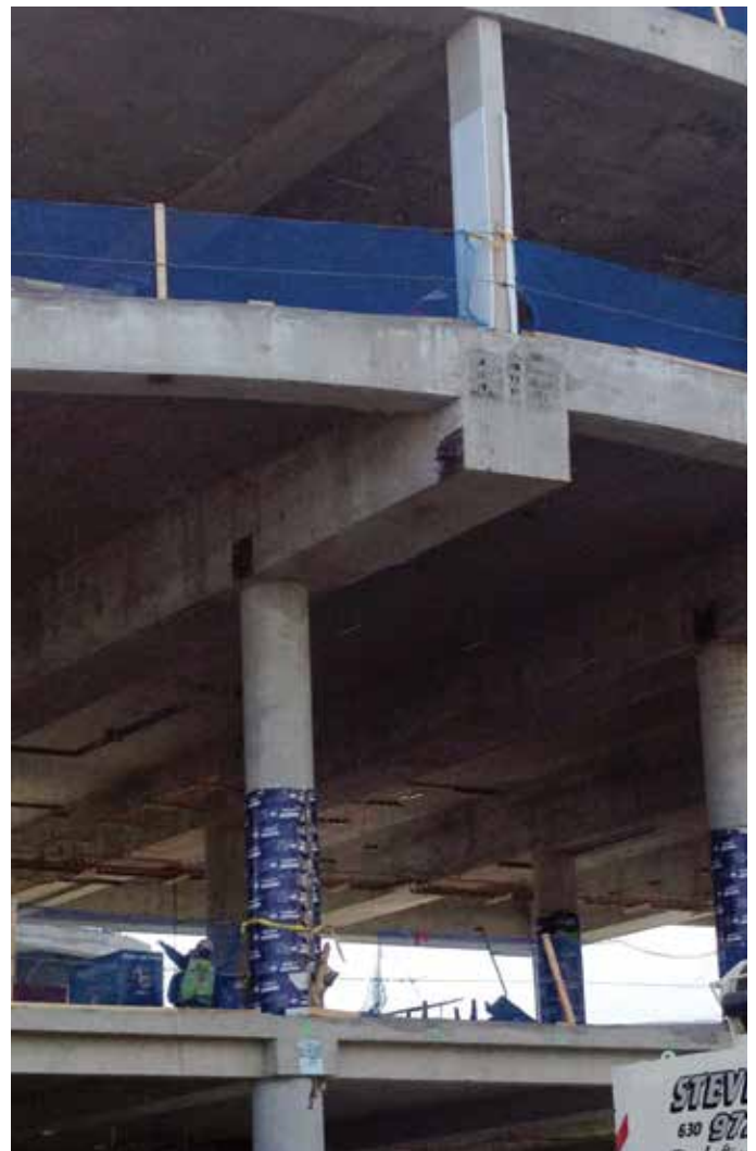
Fig. 4—Cantilevered post-tensioned transfer beam.
