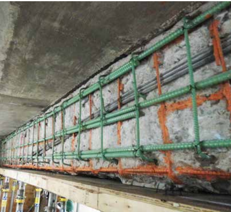
Fig. 8—Column line 9 new steel and new 0.6 in. PT cable.
