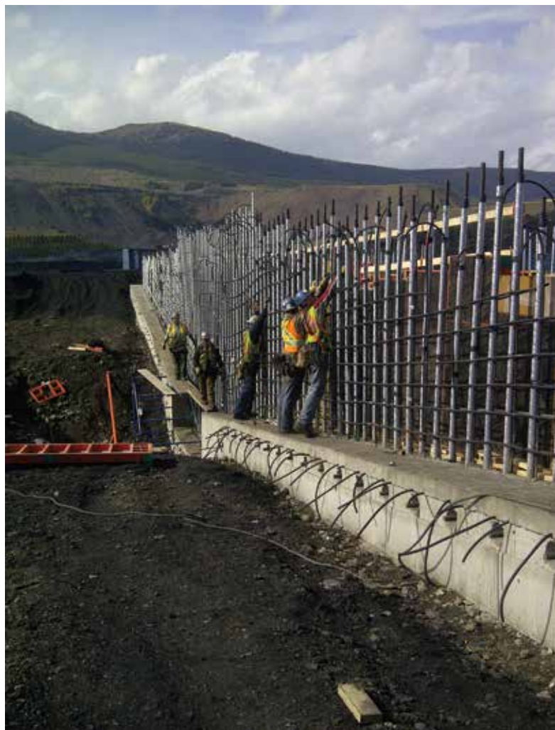
Fig. 6—Walls of tank with vertical PT bars and horizontal encapsulated unbonded tendons.
