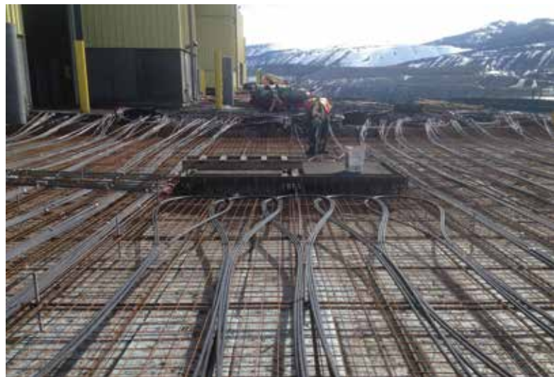
Fig. 8—Warmup slab under construction.
