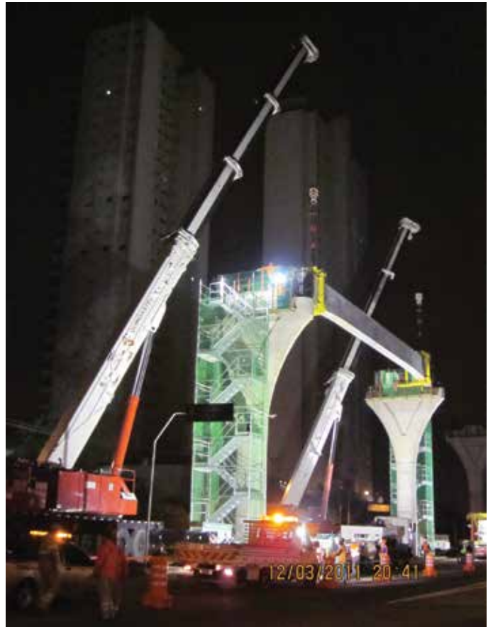
Fig. 9—Erection of PT beams.
