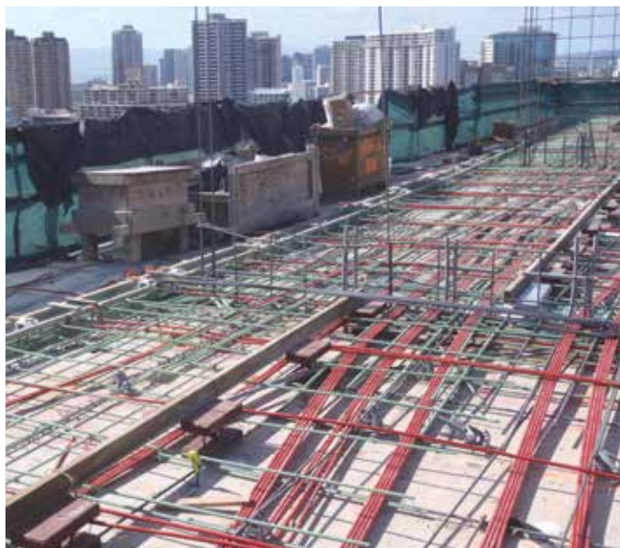
Fig. 2—PT slab under construction.
