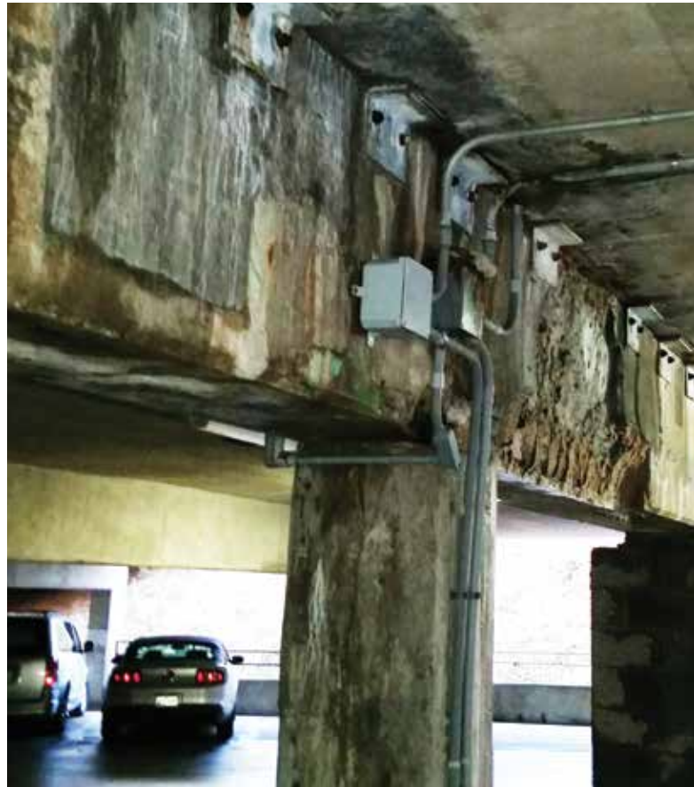
Fig. 15—Before repair, metal angles supporting slab.
