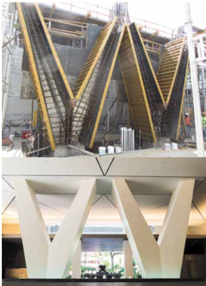
Fig. 5—W column under construction (top) and completed (bottom).
