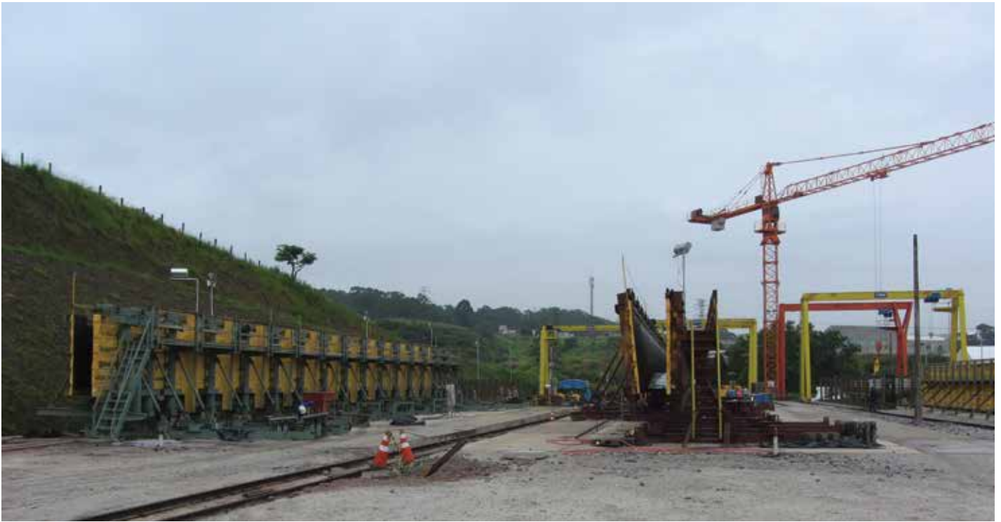
Fig. 7—Post-tensioned concrete beams in the casting yard.
