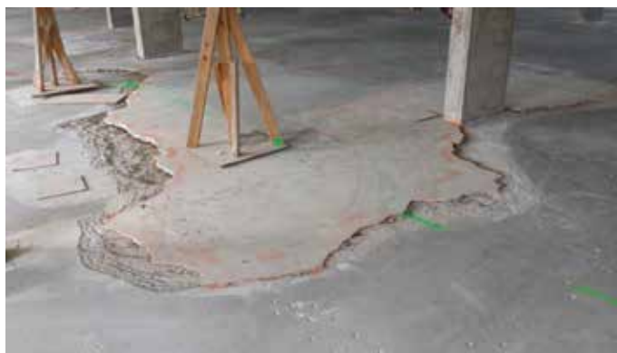
Fig. 2—Shear crack failure.
