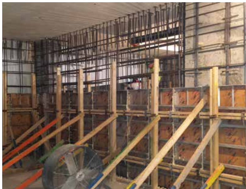
Fig. 12—Interior shear walls.
