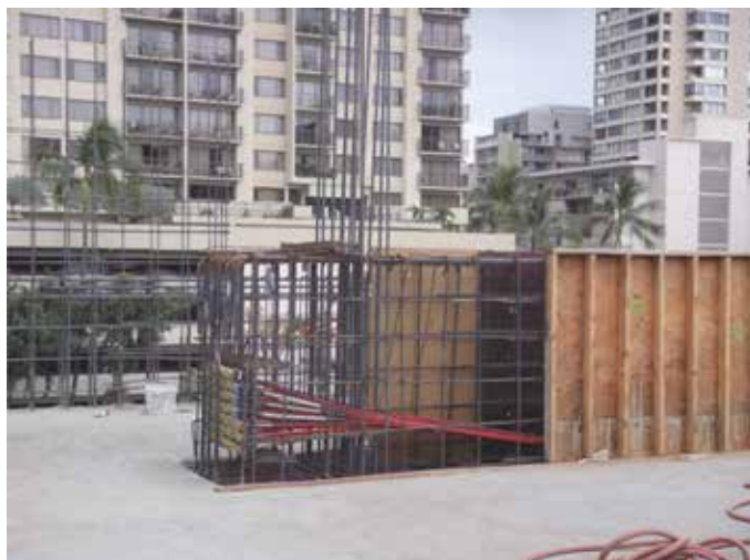
Fig. 7—PT upturn transfer girder.
