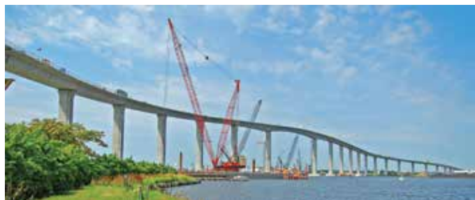
Fig. 4—Barge-mounted crane.
