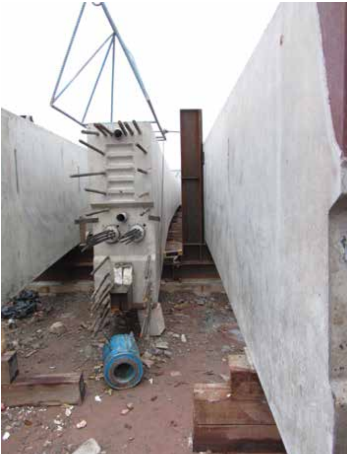
Fig. 8—Post-tensioned concrete beams at first stage stressing.
