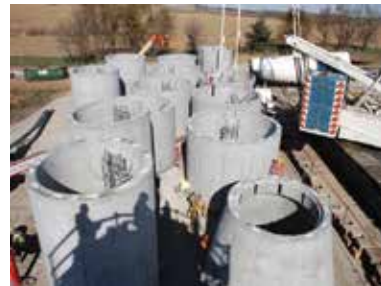
Fig. 3—Precast segments are match cast.
