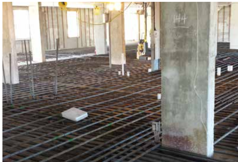
Fig. 11—Overlay reinforcement.
