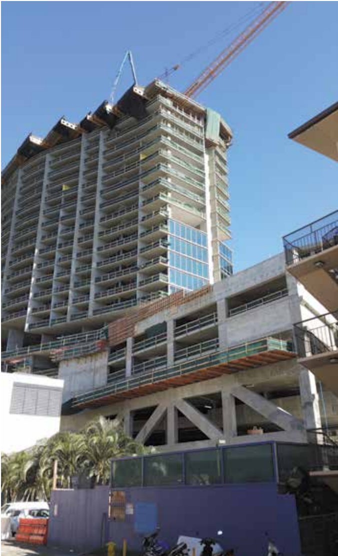
Fig. 10—PT concrete truss under construction.
