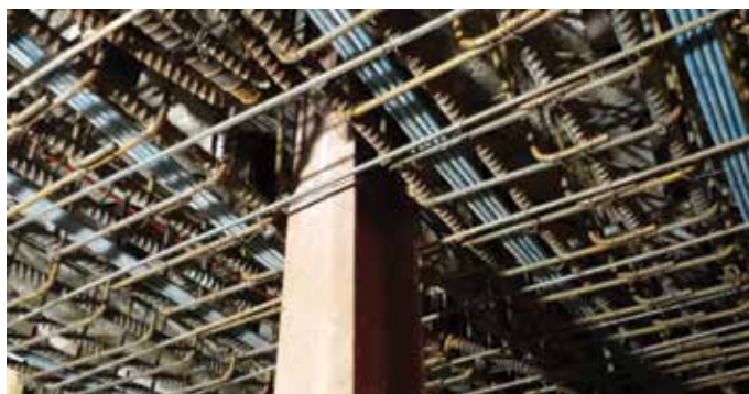
Fig. 7—Drop panels with nonprestressed and PT reinforcement.
