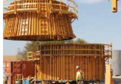
Fig. 2—On-site segment precasting.
