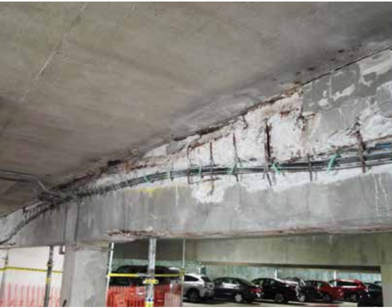
Fig. 7—Column line 9 new 0.6 in. PT cable.
