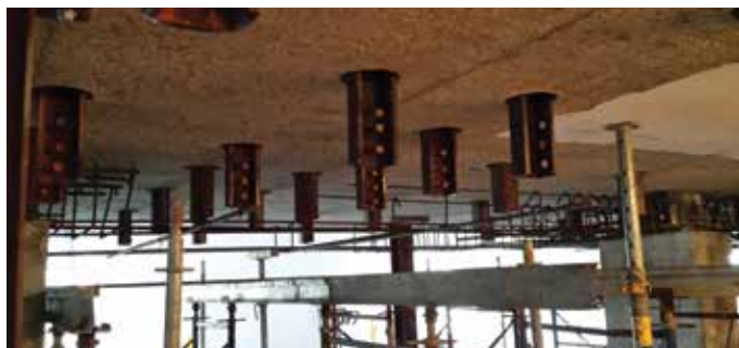
Fig. 9—Shear lugs provide continuity between drop panels and overlay slab.
