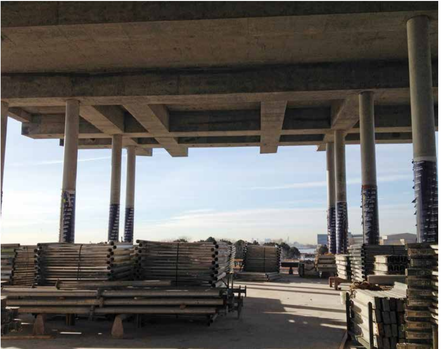
Fig. 5—Post-tensioned transfer beams.
