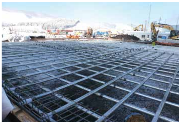
Fig. 4—Two-way grouted PT base slab.
