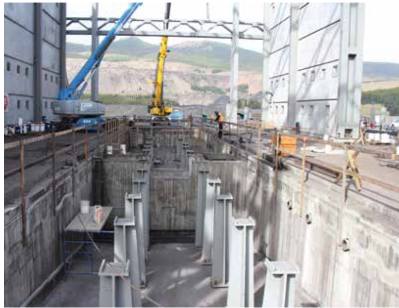
Fig. 7—Tank fully integrated with raft slab.
