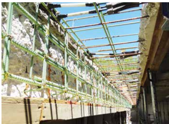
Fig. 5—Column line 15 new reinforcing bar and PT cables.
