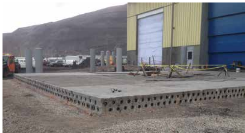
Fig. 9—Completed warmup slab.
