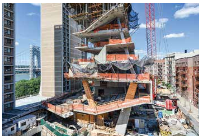
Fig. 2—Inclined columns from the foundation level up to the eighth floor.
