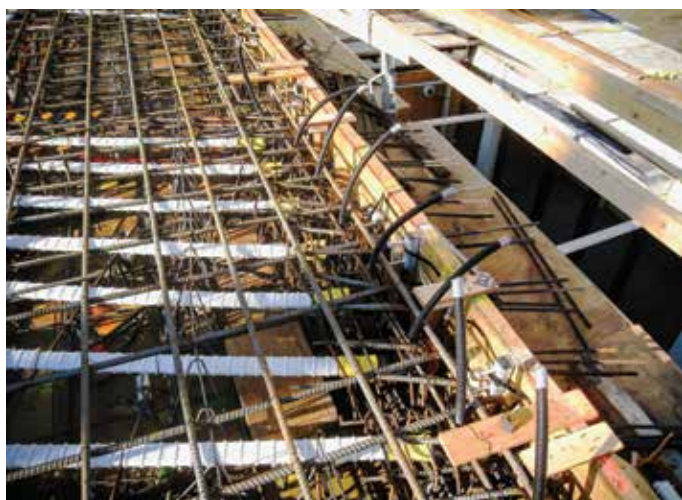
Fig. 3—Bonded post-tensioning system.
