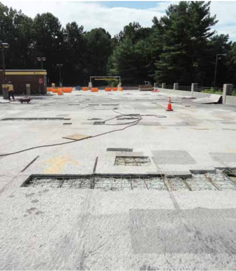
Fig. 13—Top deck PT and concrete repairs.
