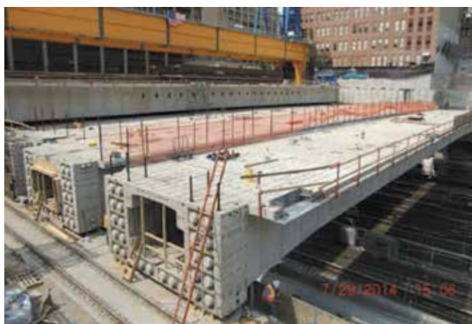
Fig. 6—Post-tensioning on face of pier segments.
