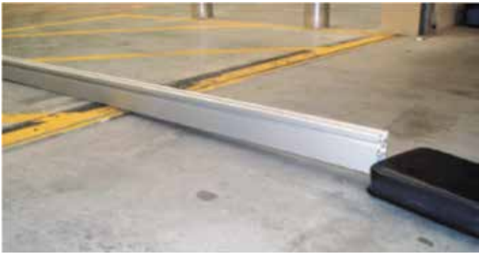
Fig. 9—Slab curl in a typical New Zealand floor.
