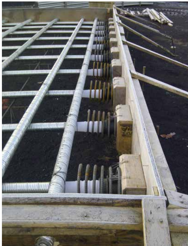
Fig. 3—Bonded PT anchorages.
