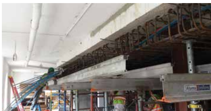
Fig. 6—Drop panels with nonprestressed and PT reinforcement.
