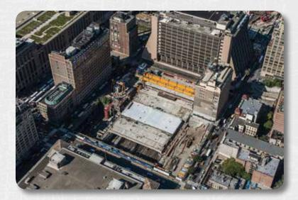
The Manhattan West Platform is a 110,000 ft<sup>2</sup> segmental post tensioned platform made of 16 adjacent bridges with a record length of 240 ft. The platform covers a 240 x 480 ft hole over active rails taking around 800,000 people a day in and out from Penn Station. Brookfield Properties is the Owner and is planning to build 7 million ft<sup>2</sup> of mixed residential and commercial use.
