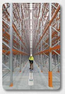
The floor was constructed as a series of large bay post-tensioned floors, coupled together so that there were only two opening joints located within the 25,000 m<sup>2</sup> (267,500 ft<sup>2</sup>) ground floor. Combined with the use of a new system for concrete floor jointing—the Rhino joint—this creates a surface that would require little to no maintenance during the life of the structure.
