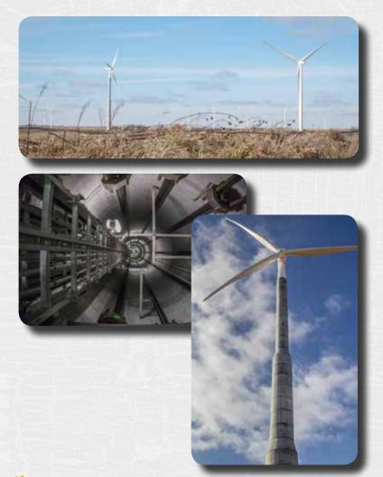
The tower is the first precast segmental concrete wind tower constructed worldwide and is the highest tower in the United States. The tower supports a Siemens 2.3 MW turbine. Also unique to the tower structure is that its segments were fully precast on site at a central casting yard, installed into the tower before being stressed in place without the use of temporary posttensioning.
