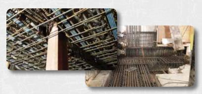
The building is a 15-story condominium with the first three levels devoted to parking. The fourth floor is designed to be a 24 in. thick column transfer slab, distributing the 12-story column loads above to the non-aligning columns below.
