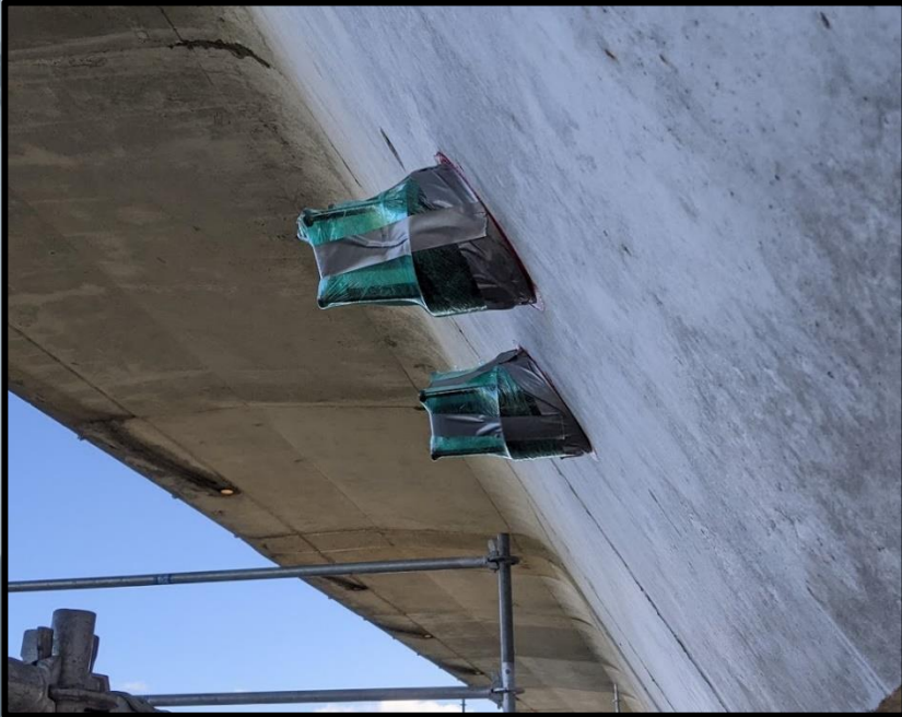
PT bar anchors on exterior face of web
