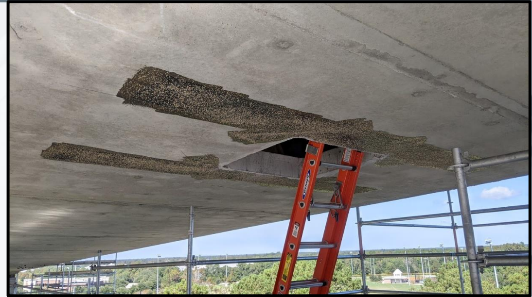
CFRP reinforcing at new access opening
