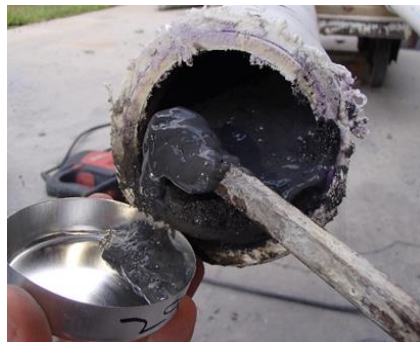
Soft grout found in MITT
