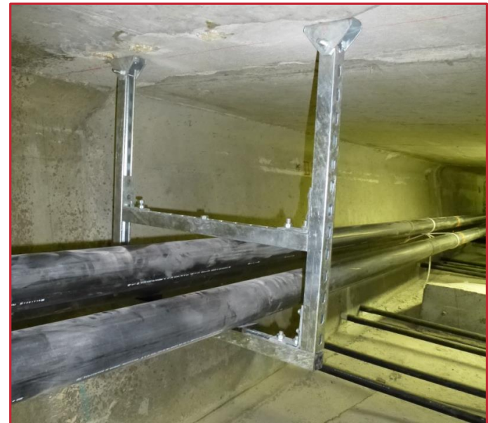
Horizontal fixation of the external tendons every 20 m
