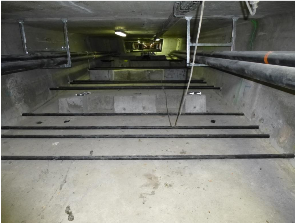
Transverse bar tendons in the inside of the box girder
