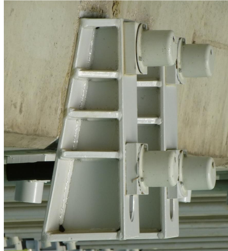
Anchorage of the bar tendon at the outside of the box girder
