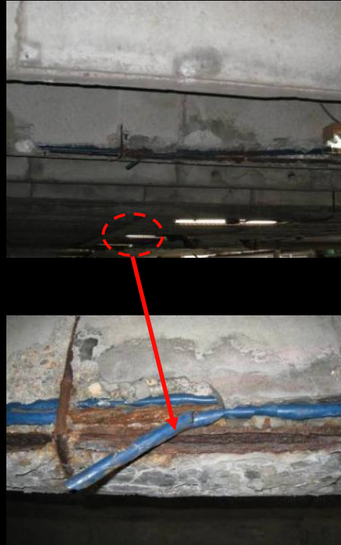
Cracking and Spalling in Overhead Concrete Pan on Roof Level
