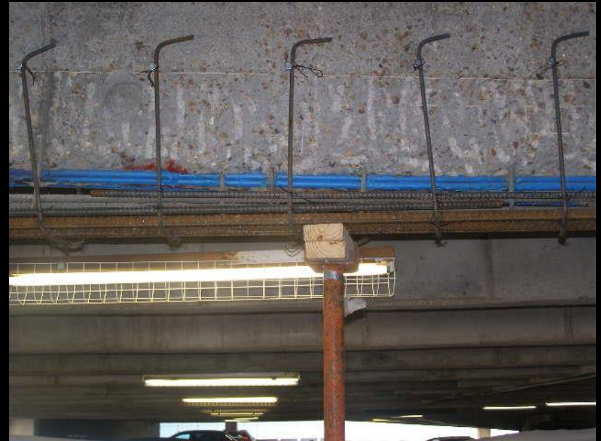
Roof Joist – Installation of Supplemental Reinforcement / Shear Connectors, Repair of PT Sheathing
