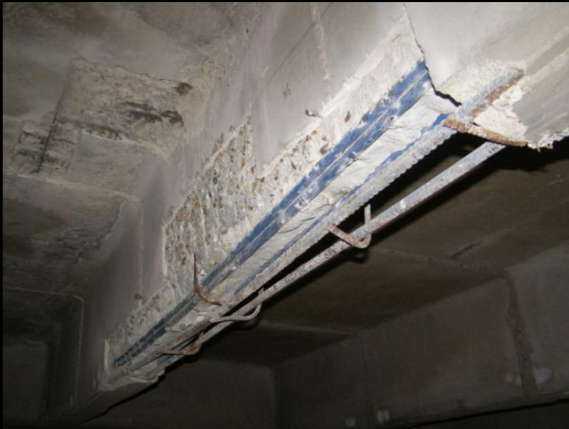
Surface Preparation for Repairs to Roof Joist
