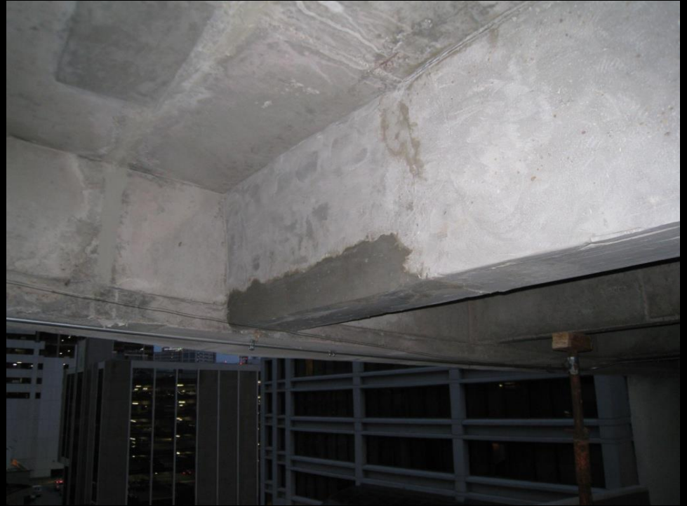
Repaired Roof Joist
