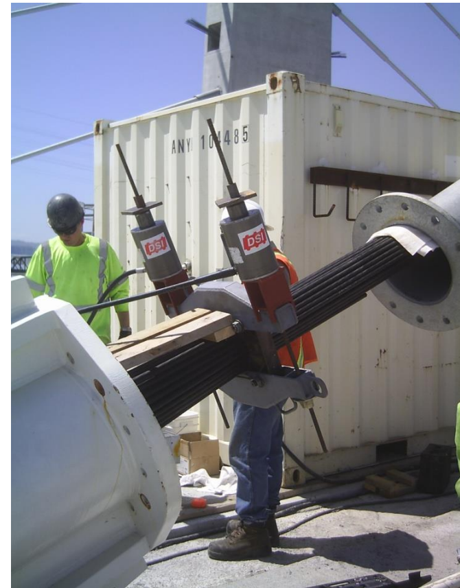
Strands compacted into hex pattern
