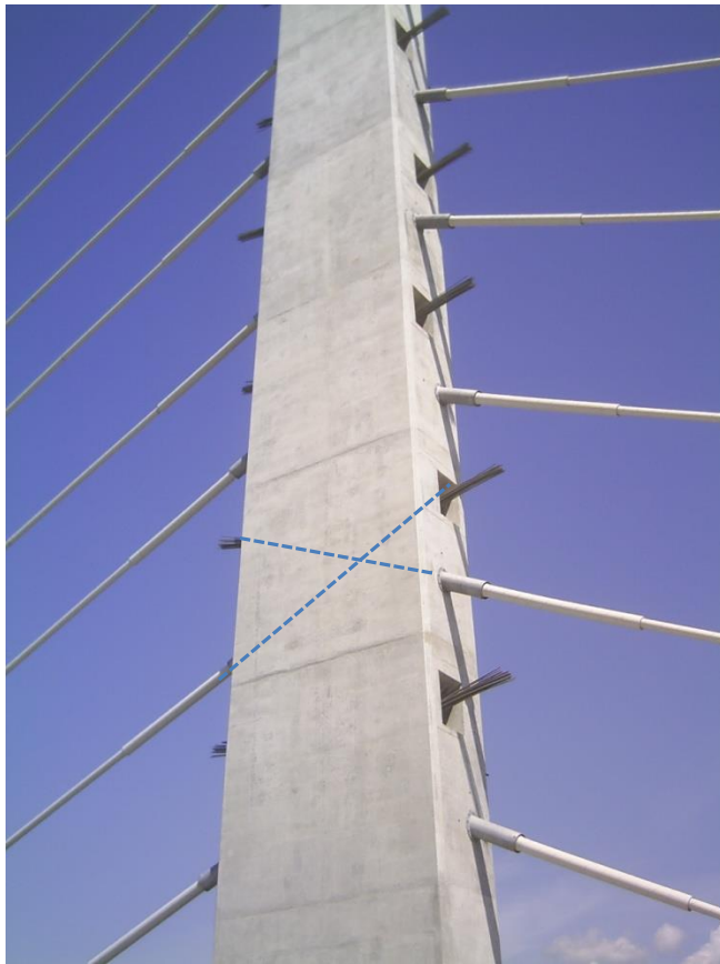
Tower showing steel Exit pipes & stressing tails
