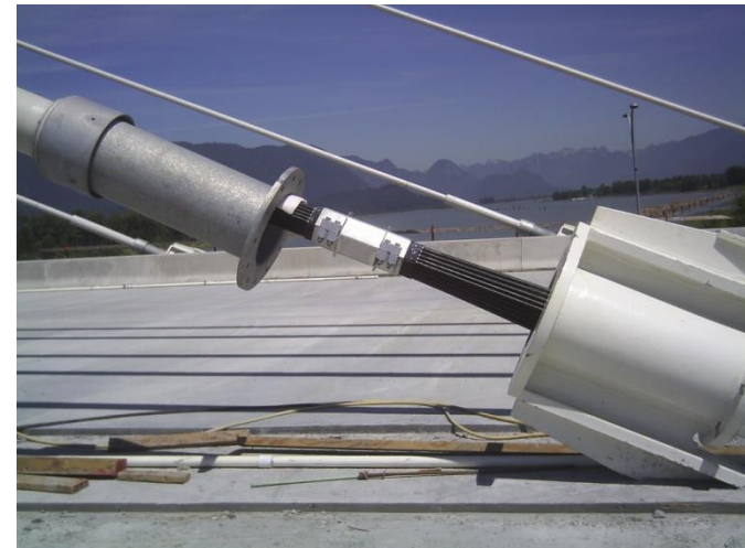
Bolted clamp- with exit and recess pipes
