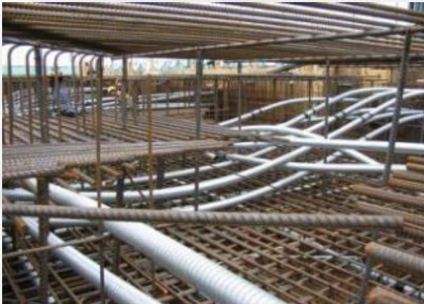
Installation of Reinforcement & Tendon
