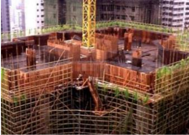
Installation of Side Formwork
