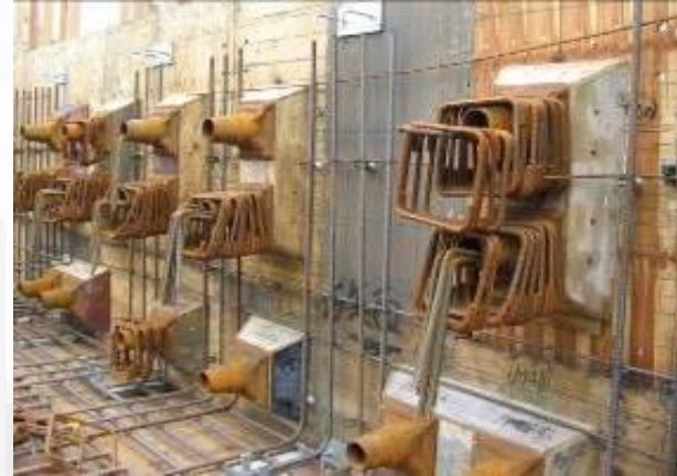
Installation of Anchorage
