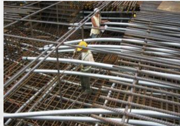
Installation of Reinforcement & Tendon
