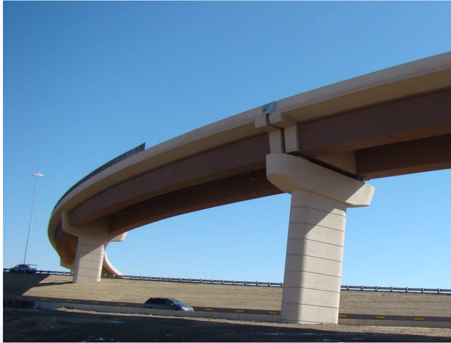
84" Curved U Girders, 3 Units, 10 Spans 230' Main Span over IH70, 800' Radius Completed in 2008
