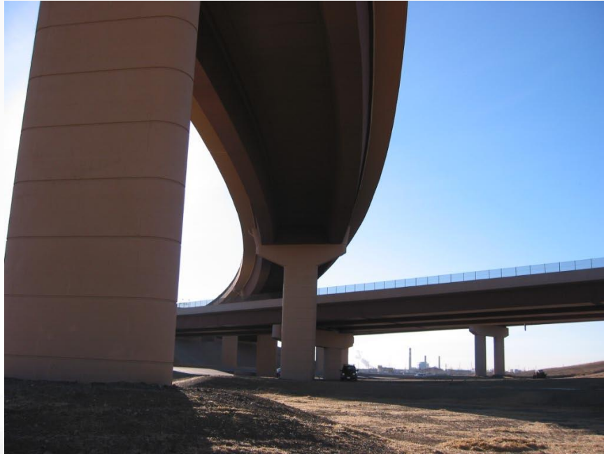
84" Curved U Girders, 2 Units, 12 Spans 230' Span Lengths, 765' Radius, 38' Deck Completed in 2005
