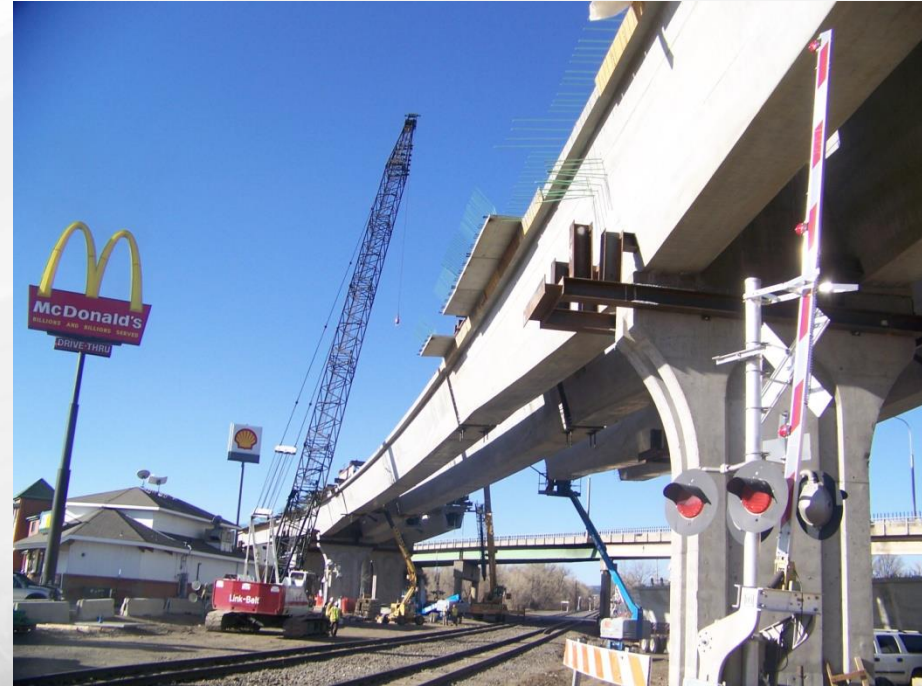
84" Straight and Curved U Girders, 2 Phase Project 256' Main Span over UPRR, 1200' Radius Completed 2009
