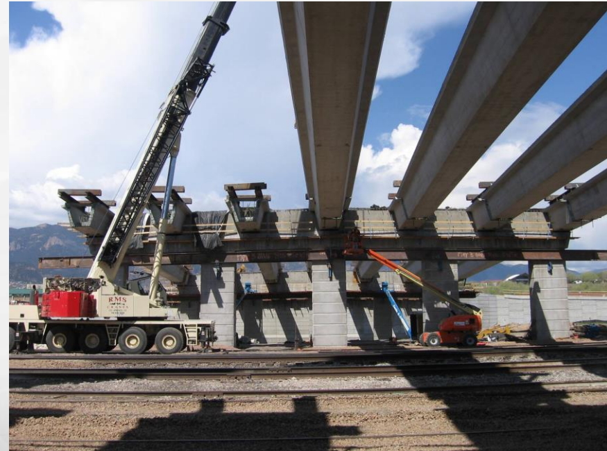
60" Straight U Girders, 4 Spans 150' Main Span over UPRR, Constructed without Shoring Completed 2005
