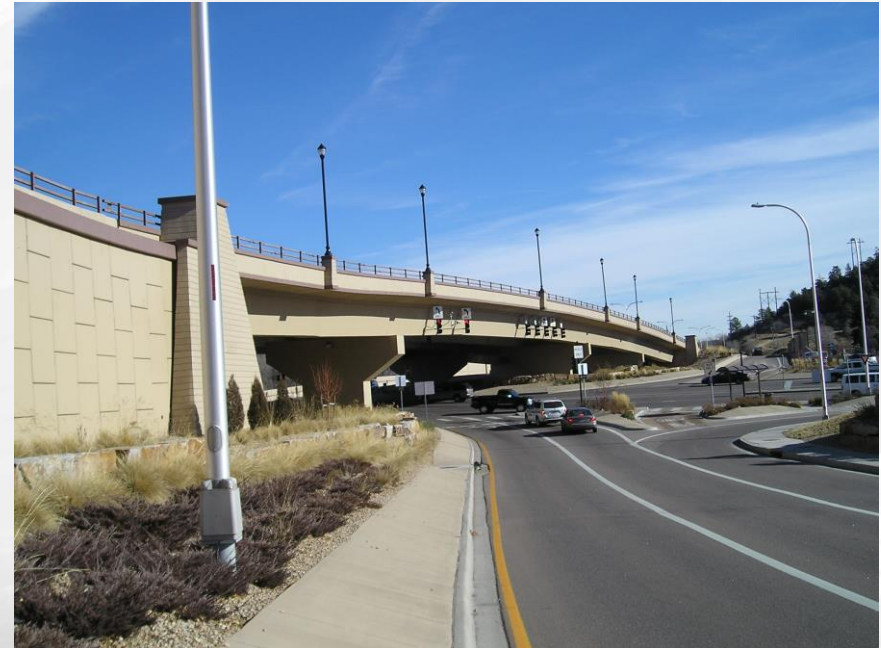
84" Curved and Straight U Girders, 4 Spans 220' Main Span, 700' Radius, 98' Deck Completed 2008
