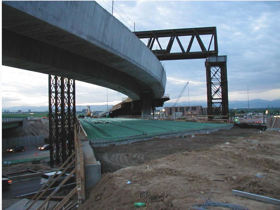
84" Curved U Girders, 8 Spans 250' Main Span, 750' Radius Completed in 2000
