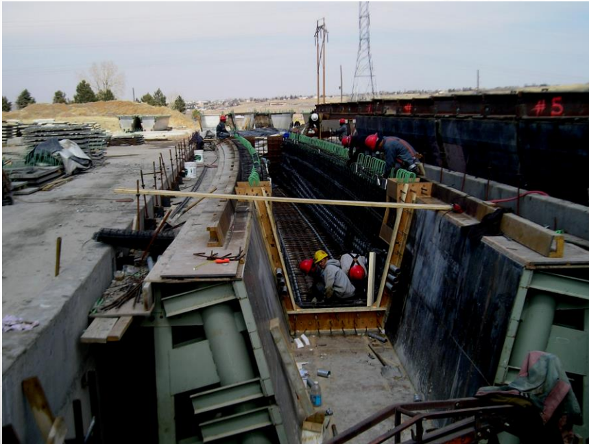
Girder Casting Yard and Forms
