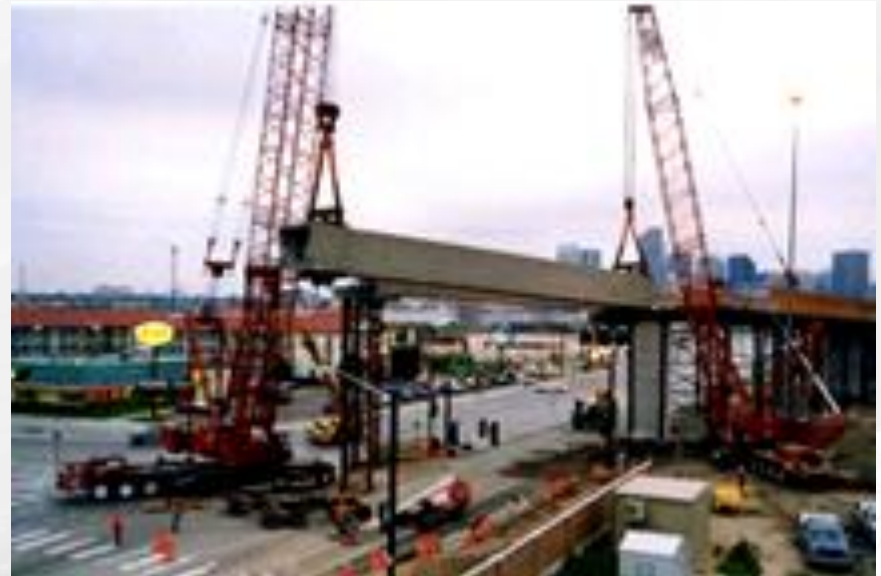
96" Straight U Girders, 6 Spans 230' Main Span over IH25, Site Cast Precast Girders Completed 1998
