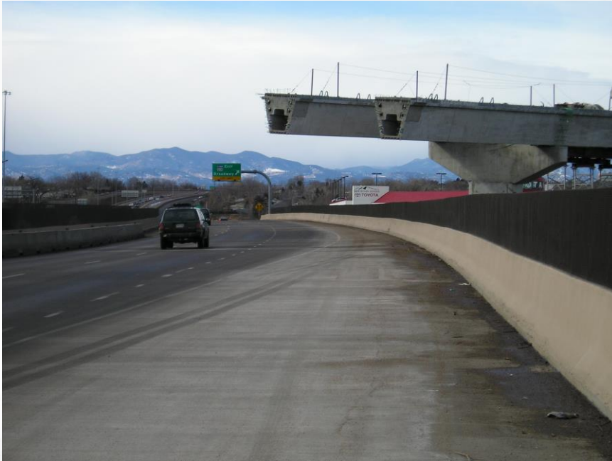
84" Curved U Girders, 8 Spans 200' Span Length, 800' Radius Completed in 2005
