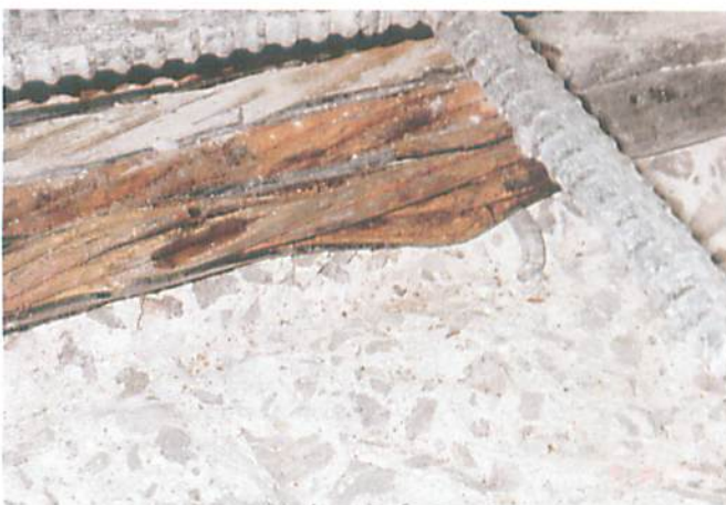
Fig. 1 - Corroded strands exposed for visual inspection
