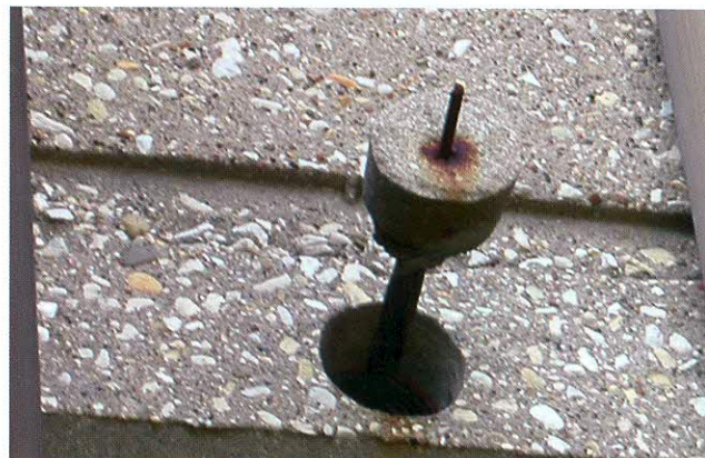
Fig. 1 – Visual Indication of a Broken Tendon
