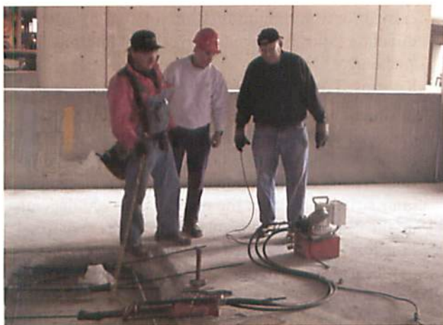
Fig. 11 – Stressing of Tendon at Intermediate Stressing Anchor
