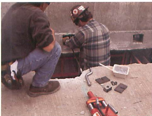
Fig. 19 – Installation of Split Anchors
