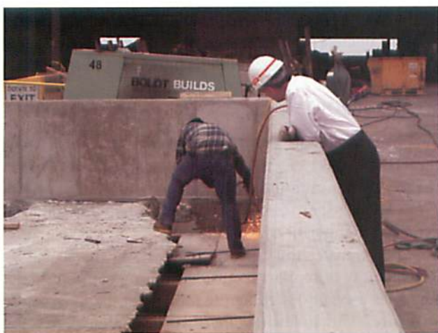
Fig. 21 – Detensioning Tendons by Heating with a Torch
