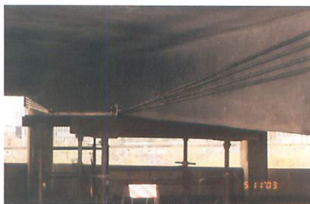
Fig. 27 – Deviated Beam Strengthening Tendons
