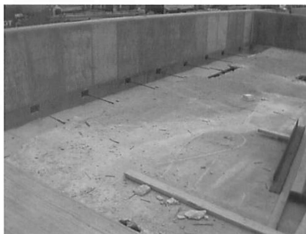
Fig. 18 – New Perimeter Beam at the Edge of Opening
