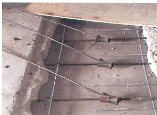
Fig. 10 – Intermediate Stressing Anchors for Slab Repair
