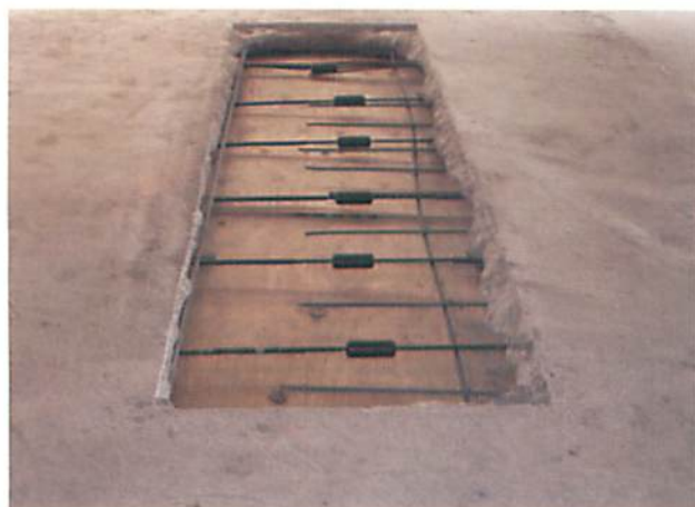
Fig. 9 – Couplers for Slab Repair
