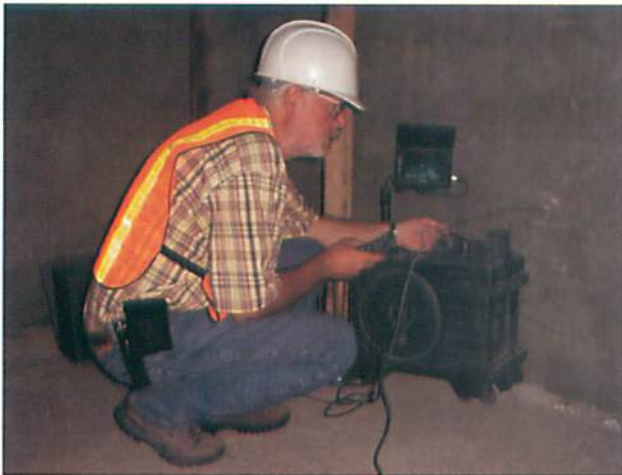
Fig. 3 – Videoscope Inspection of Post-Tensioning Tendon
