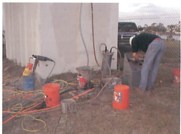
Fig. 5 – Vacuum Grouting Operation
