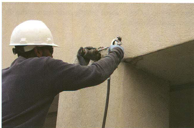
Fig 15 - Grease injection at anchorages
