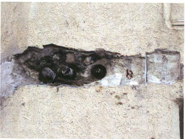
Fig. 8 - Deteriorated anchorages due to improper end-cap installation
