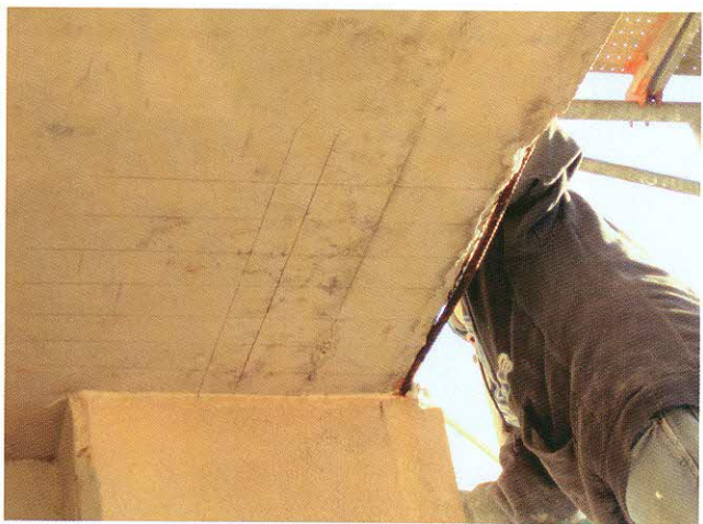
Fig. 5 - Marked tendons at the soffit of slab
