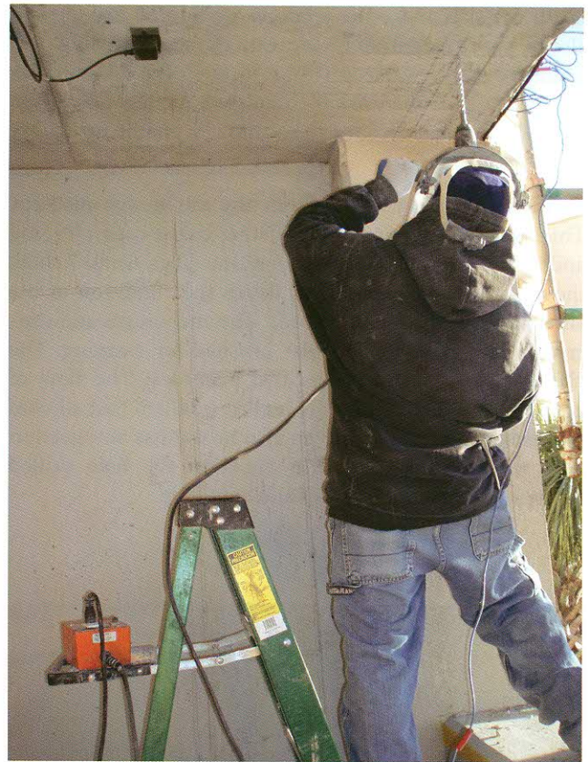
Fig. 11 - Drilling through slab and tendon sheathing
