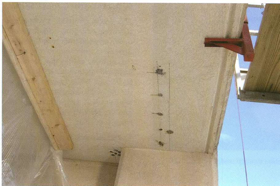
Fig. 13 - Drilled holes into tendon sheathing at balcony
