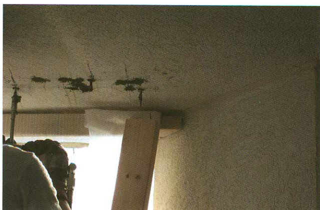
Fig 14 - Injecting grease from ports located underneath the slab
