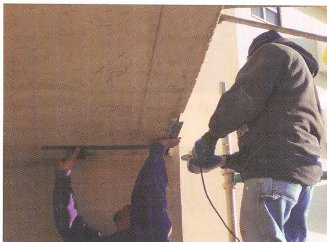
Fig. 4 - Marking of tendons
