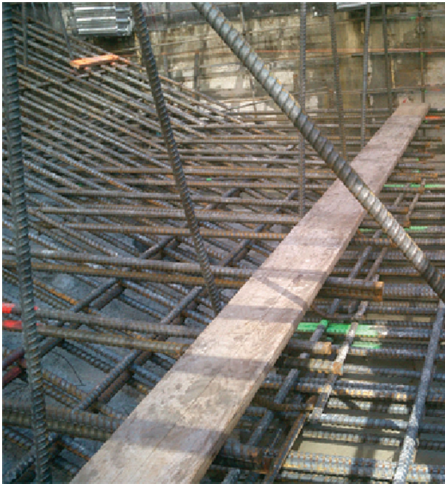
Fig. 7—Construction of mat foundation. (Photo courtesy of Cary Kopczynski & Company.)
