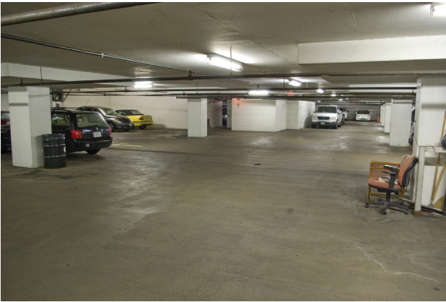
Fig. 3—The floor of the second basement is actually the top surface of the foundation. Forty years after construction, it is crack-free, watertight, and completely dry. The 10 in. (250 mm) thick drop panels of the first basement deck are clearly visible in the ceiling of this photo: they resemble broad soffits surrounding the load-bearing pillars. (Photo by Steven H. Miller, courtesy of CTS Cement Manufacturing.)
