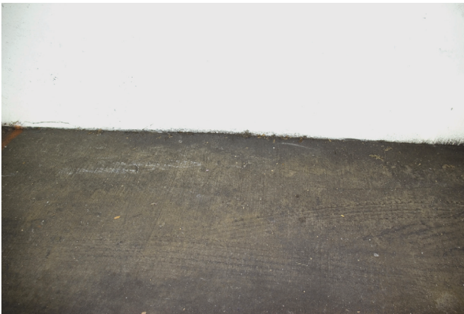
Fig. 4—Even at the meeting point of foundation and basement wall, there is no evidence of cracking or leakage. (Photo by Steven H. Miller, courtesy of CTS Cement Manufacturing.)
