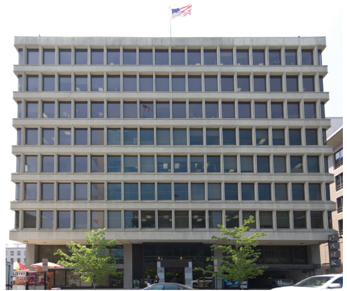
Fig. 5—Forty years later, the building is stable and in excellent condition. The thin deck-slabs made possible by post-tensioning allowed the designers to get an extra story into the structure and still stay under the city's absolute height limit. The building is currently occupied by offices of the Federal Bureau of Prisons. (Photo by Steven H. Miller, courtesy of CTS Cement Manufacturing.)
