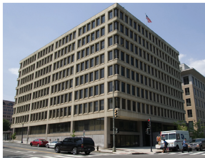
Fig. 1—500 First Street, NW is an eight-story building with two basement levels. Like many sites in the Washington, DC, area, there were significant groundwater issues to contend with in constructing the foundation. Erected in 1967, it was the first building in the city constructed with post-tensioning. (Photo by Steven H. Miller, courtesy of CTS Cement Manufacturing.)
