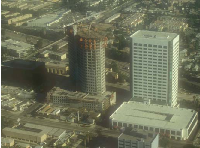
Fig. 4—The Tower under construction.
