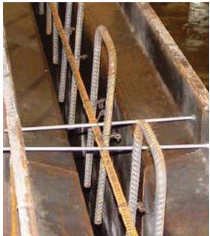
Fig. 6—U-bar positioning and form ties.
