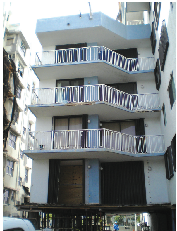
East face (note spalls evident on balcony edge).
