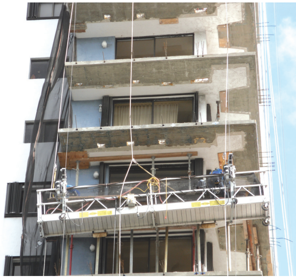
East face formwork removed, concrete placed.
