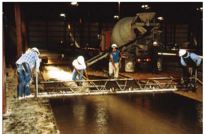
Fig. 6—Concrete placement.
