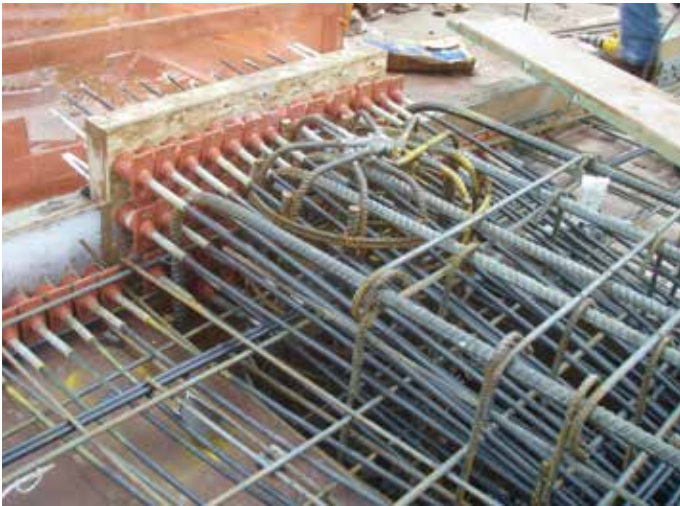
Fig. 3—Unbonded post-tensioned wide beam-slab-column connection. (Photo: Cary Kopczynski & Company)
