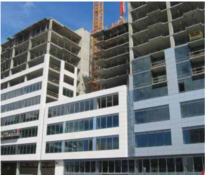
Fig. 2—Case study building under construction.
