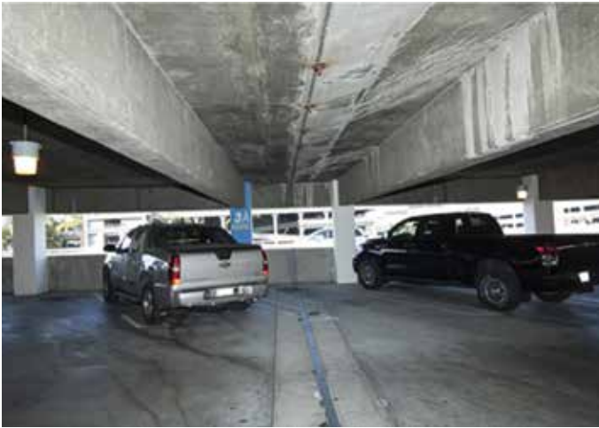
Fig. 5—East/west expansion joint.
