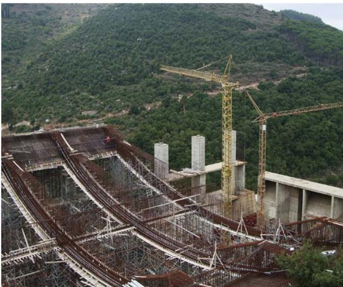
Fig. 9—Transverse beams to provide lateral resistance
