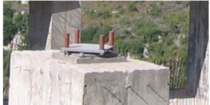
Fig. 8—CCL PG Guided Temporary Sliding Bearing.
