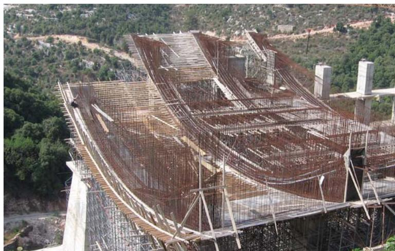
Fig. 1—One-way slab roof.
