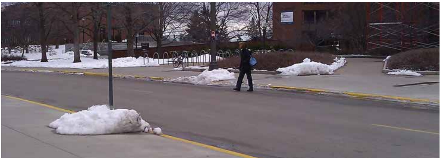
Fig. 2—Finished joint free pavement.
