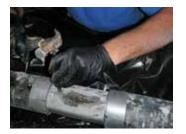
Fig. 14—Chipping grout to expose strands and observe level of saturation with corrosioninhibiting impregnation material.
