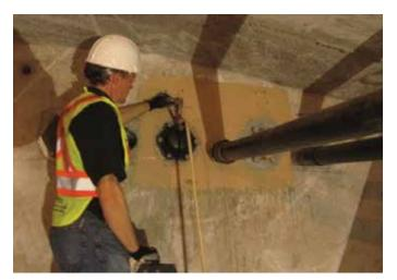
Fig. 10—Impregnation being completed from end of tendon.
