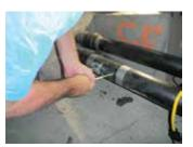
Fig. 12—Removal of plastic duct after cutting.
