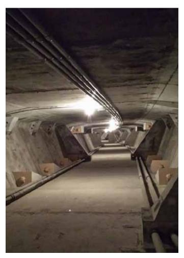
Fig. 9—FDOT cable impregnation trial bridge interior view. External tendons visible along bottom of box section.
