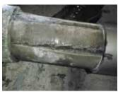
Fig. 13—Exposed grout condition after removal of duct. Impregnation material visible.
