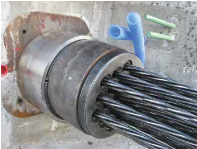
Fig. 10—Rib tendon anchorage with detensioning hardware.
