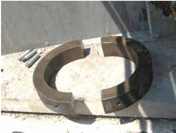
Fig. 11—Detensioning shims.
