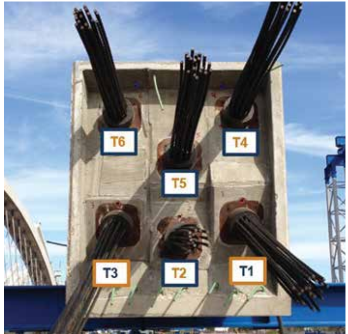
Fig. 8—Tendon anchorage locations.
