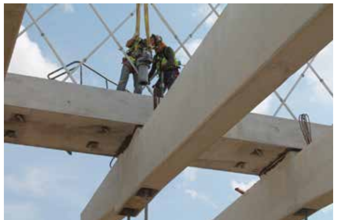
Fig. 7—Arch-to-floor beam connection.
