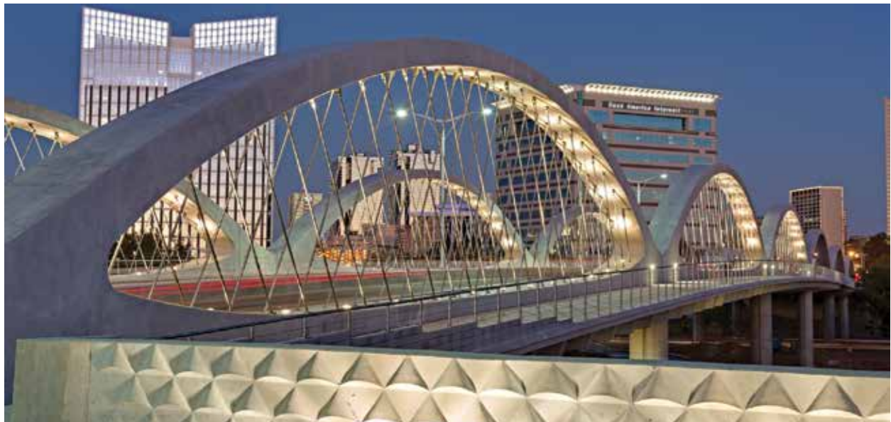
Fig. 1—Photograph of West 7th Street Bridge looking toward downtown. Photo courtesy of Liam Frederick.
