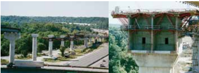
Fig. 8—External tendons in precast segments (left) and internal tendons in cast-in-place segments (right) in 895 interchange.
