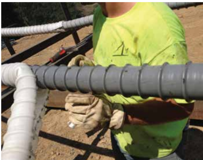
Grout 3 tendon is fully grouted.
