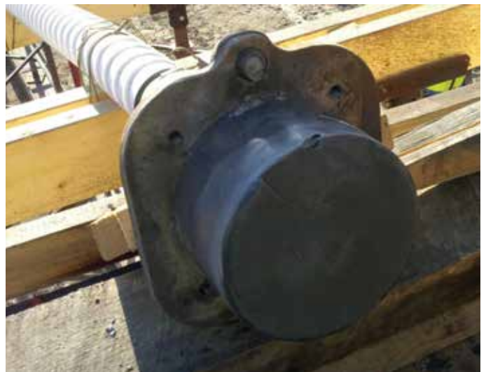
Grout 3 outlet end cap fully grouted.
