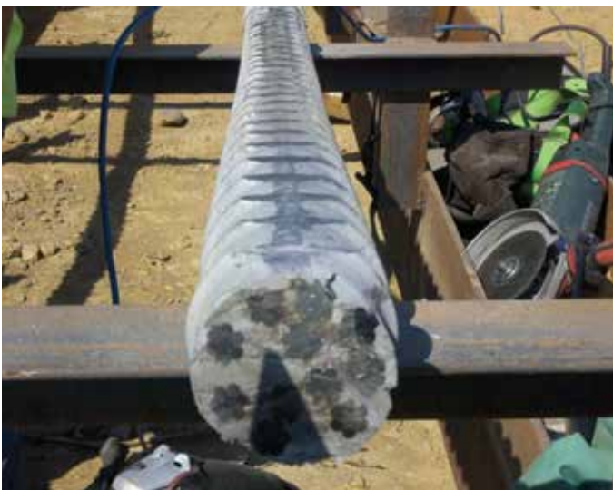
Grout 2 tendon has void along top.
