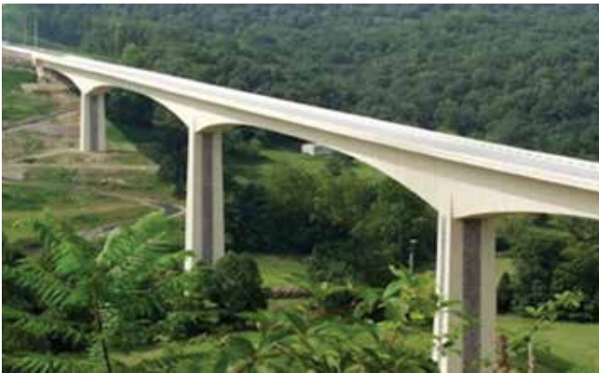
Fig. 7—Cast-in-place segmental bridge on Smart Road near Blacksburg, VA.
