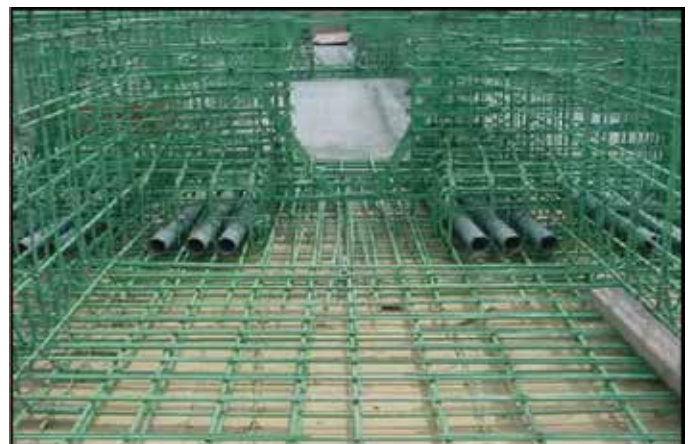
Fig. 2—Deviation saddle and bottom slab reinforcement.
