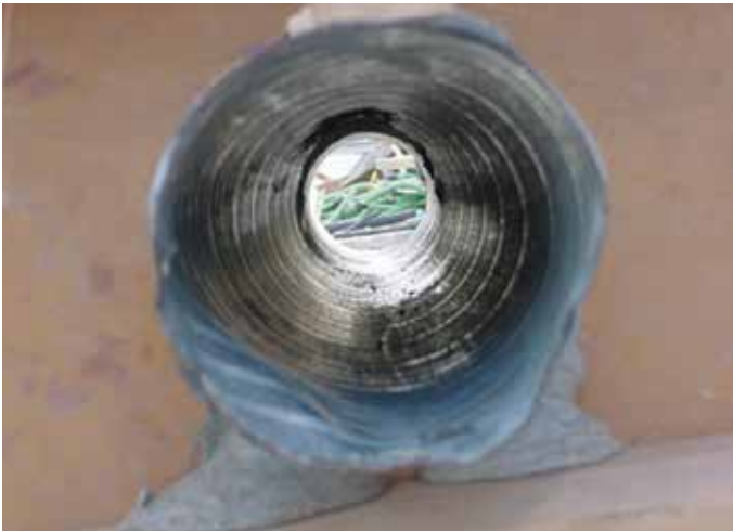
Fig. 14—Interior of PT corrugated duct after using mandrels.
