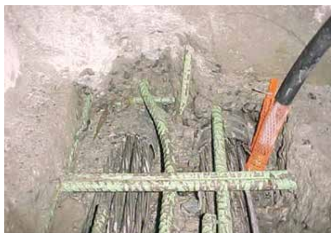
Fig. 10—Hydroblasting grout from around strands in bottom slab.
