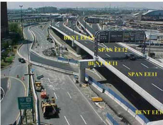
Fig. 15—View of terminal-area roadway viaducts, Spans EE11 and EE12.
