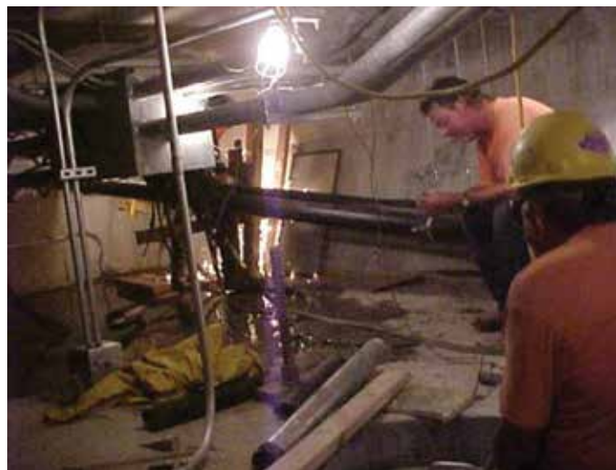
Fig. 6—Removing HDPE duct around strands and installing clamps.
