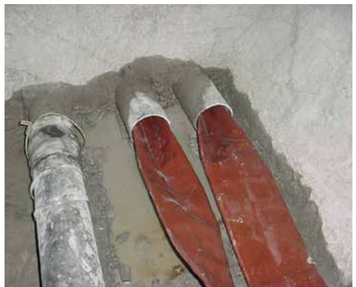
Fig. 11—Inserting inflatable tubes (mandrels) into bent steel pipes.
