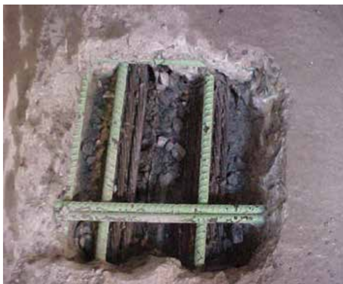
Fig. 7—Exposing strands in portion of tendon embedded in bottom slab.
