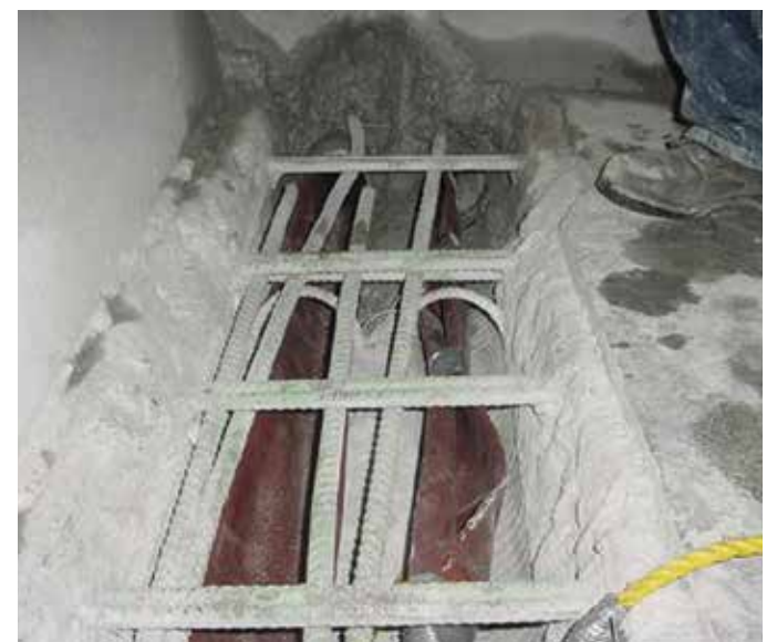
Fig. 12—Inserting inflatable mandrels in cleaned ducts path in bottom slab.
