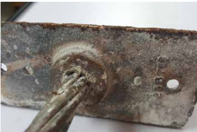
Fig. 19—Specimen No. 5: anchor, bearing side.
