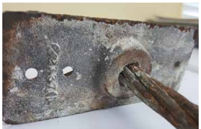
Fig. 17—Specimen No. 4: anchor, bearing side.
