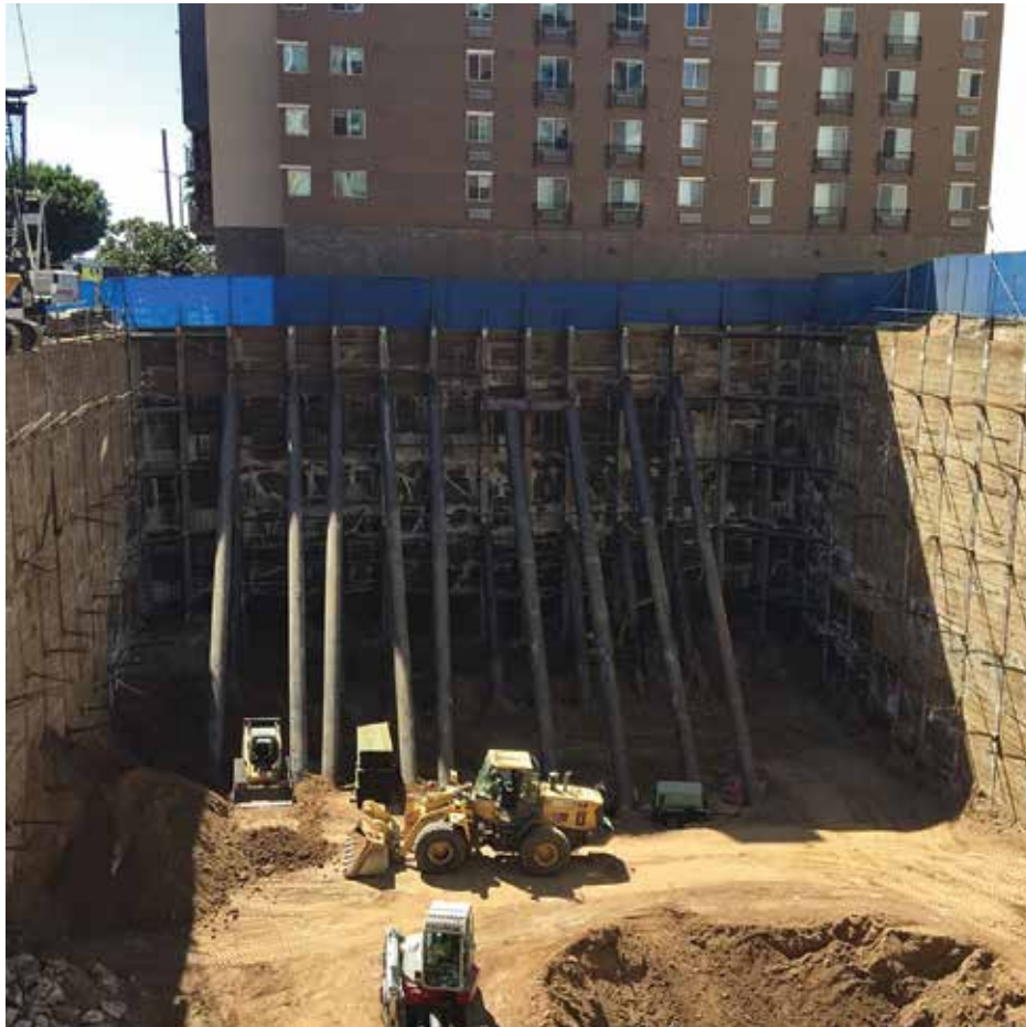
Fig. 2—Deep basement temporary shoring.
