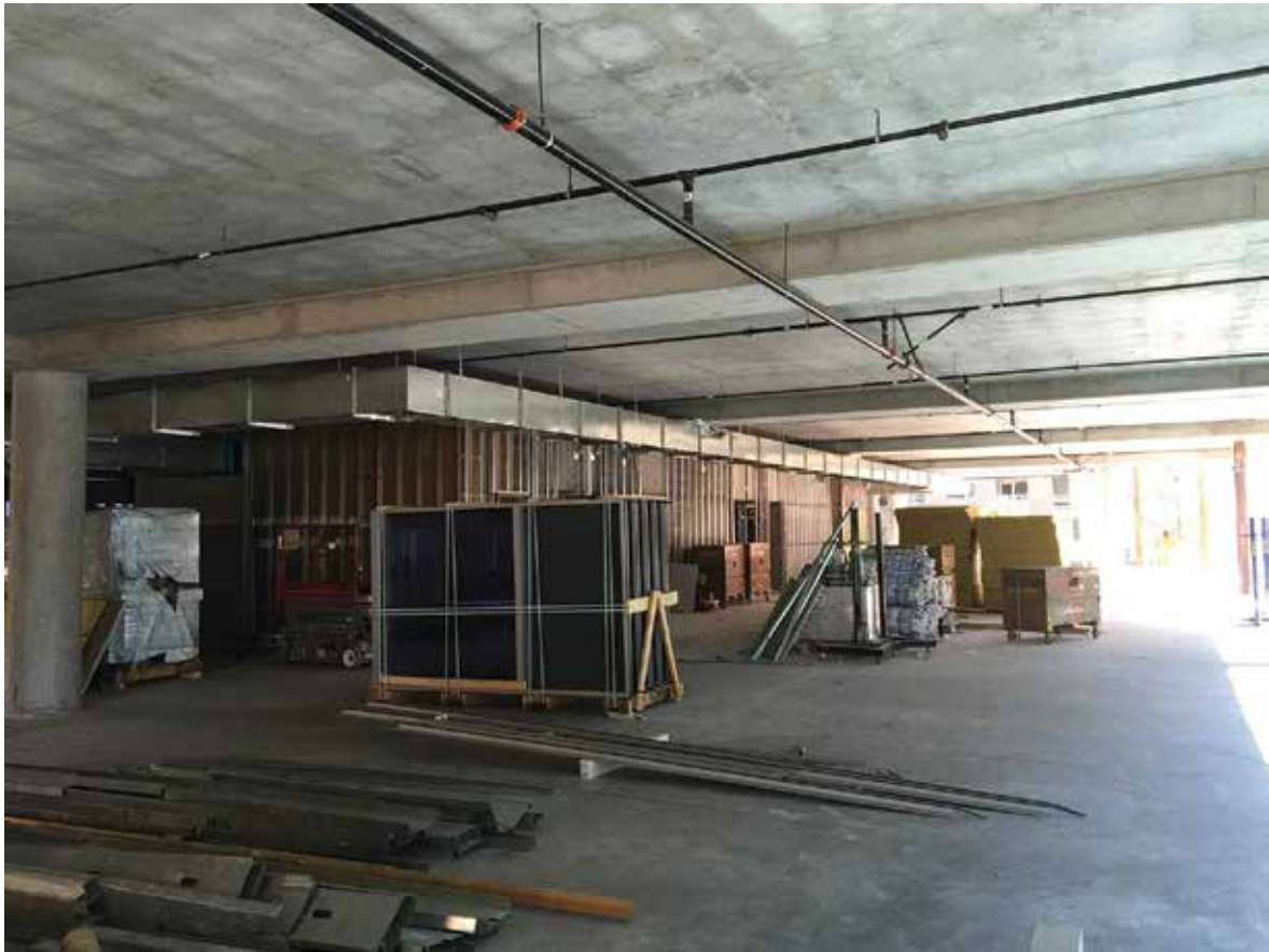
Fig. 4—Long-span framing system at office floors.
