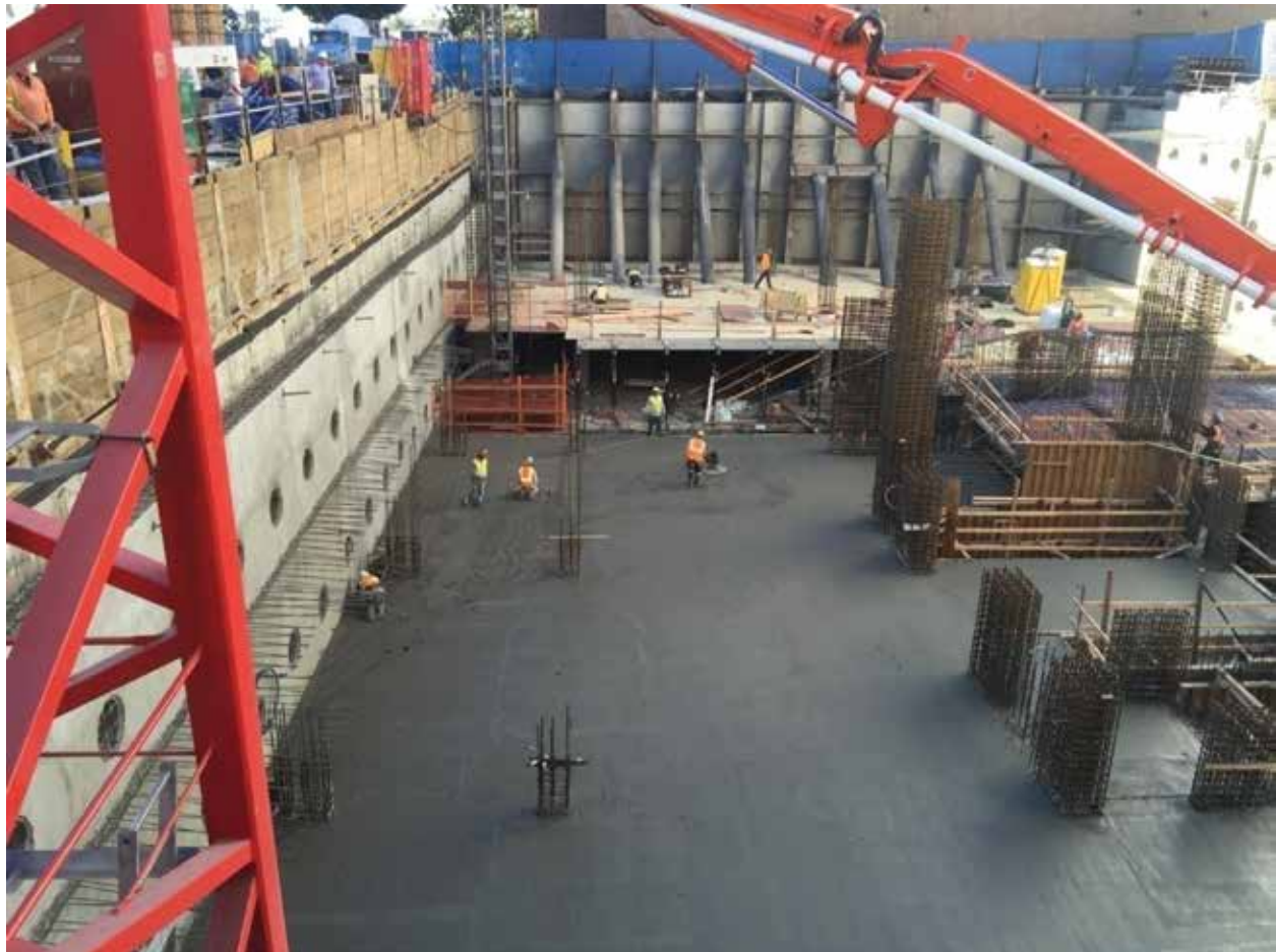
Fig. 3— Basement wall installed against temporary shoring in advance of floor slabs.
