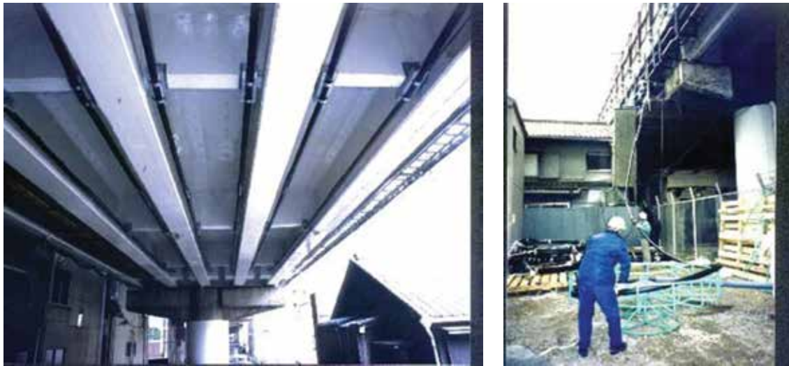
Fig. 5—Hanshin Expressway underneath view and installation in a limited area.
