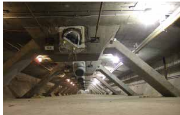
Inside of the bridge
