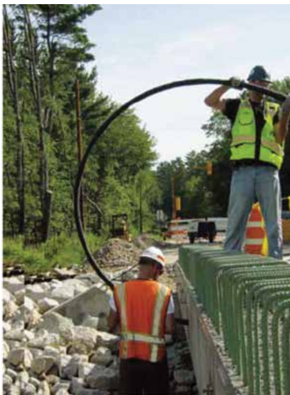
Passing CFCC strand through duct
