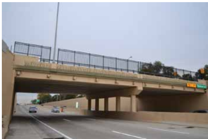
Pembroke bridge over Southfield Freeway
