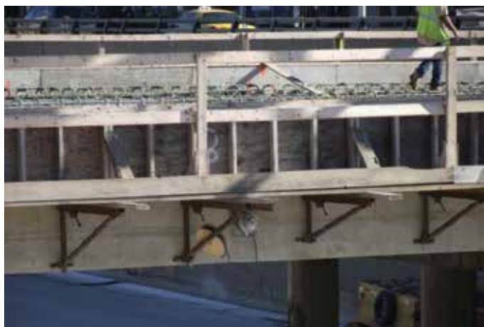
End of post-tensioning strands
