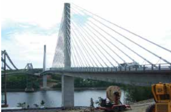
Appearance of the bridge
