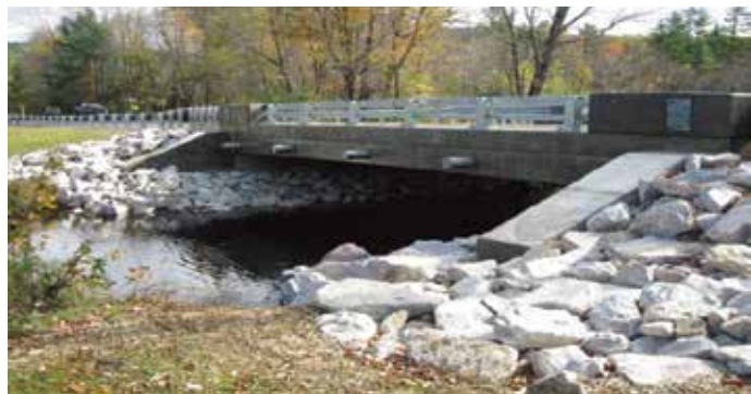
Side view of the bridge with the ends
