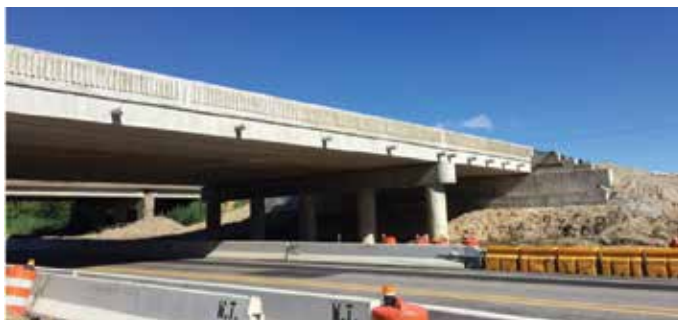
Side view of the Bridge with the ends of CFCC strands
