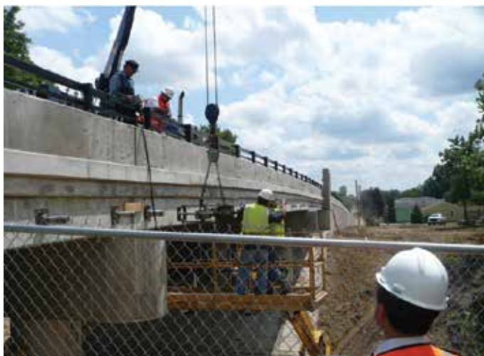
Post-tensioning of CFCC strand using the same equipment as steel strands
