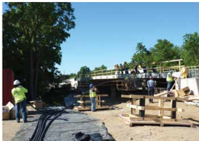
Passing CFCC strand through a duct
