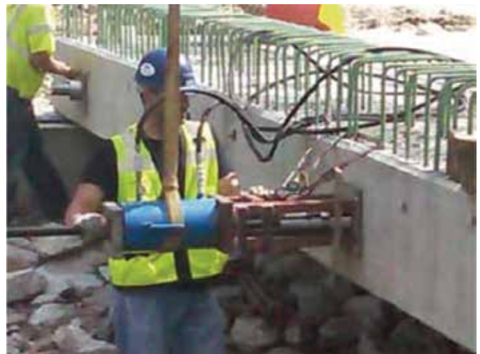
Post-tensioning of CFCC strand
