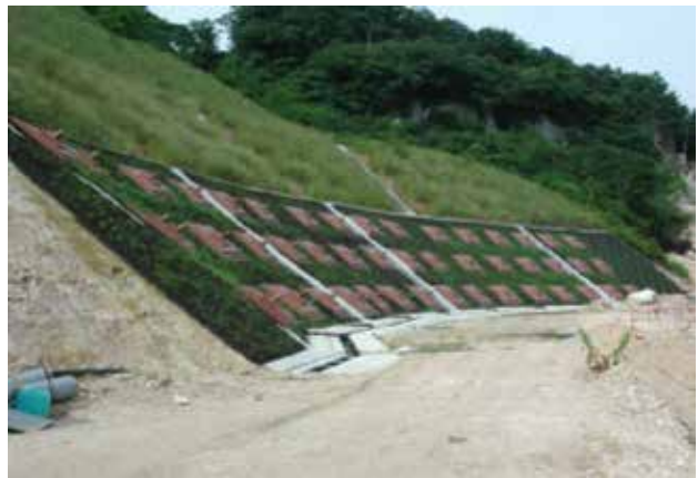
Fig. 13— In hot spring areas, due to the strong acid-related environment, steel materials are unusable.
