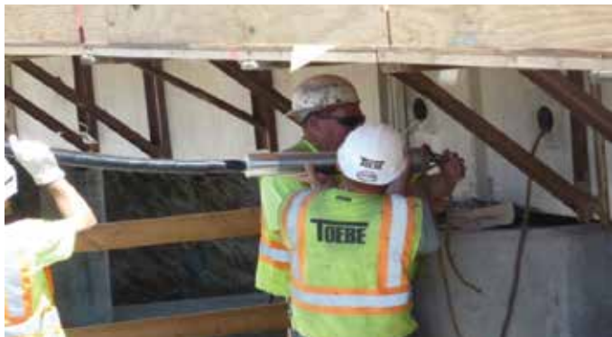
Passing CFCC strand through a duct
