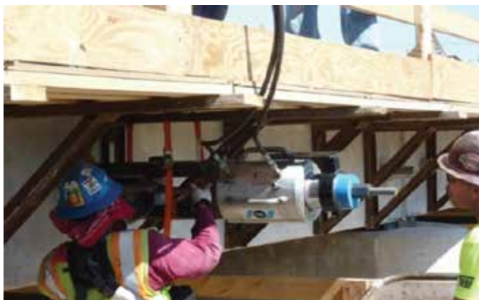
Post-tensioning of CFCC strand
