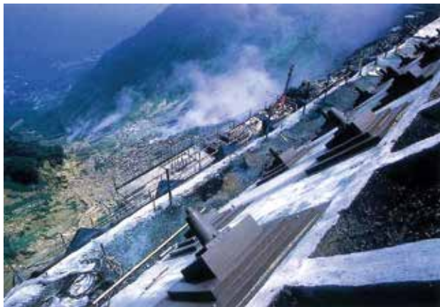
Fig. 13— In hot spring areas, due to the strong acid-related environment, steel materials are unusable.
