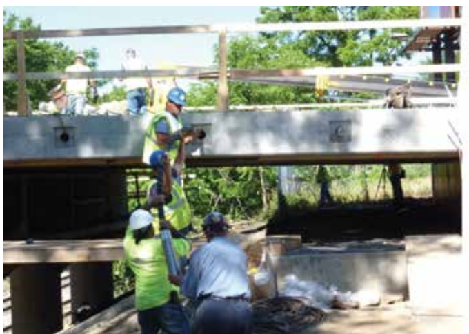
Passing CFCC strand through a duct
