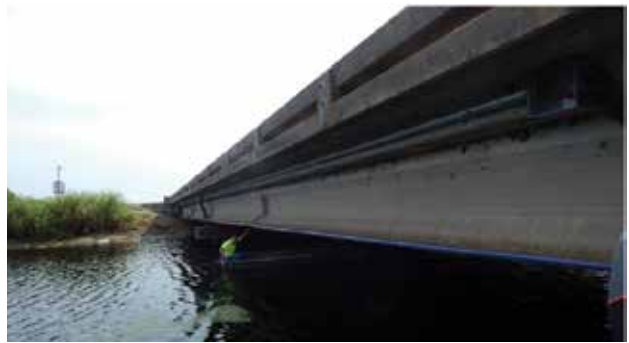
Side view of the bridge and post-tensioning cable
