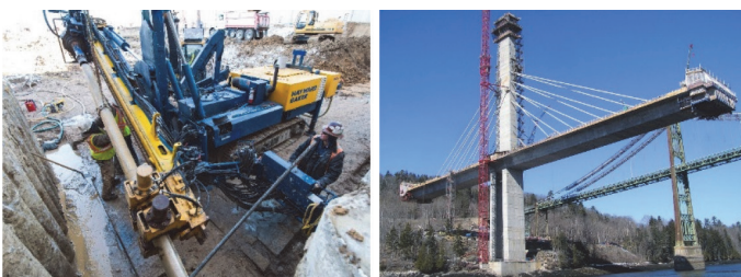
Fig. 7—Bonded PT used in earthwork and cable-stayed bridge applications.
