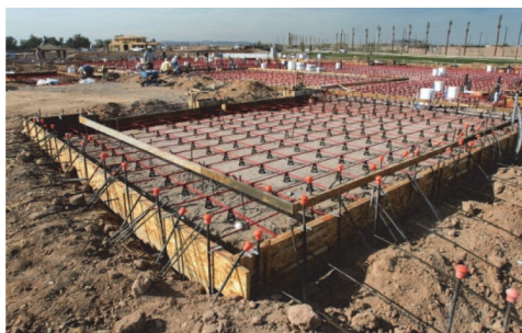
Fig. 6—PT slab-on-ground foundation.
