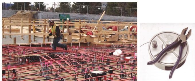
Fig. 11—Installation of PT system.
