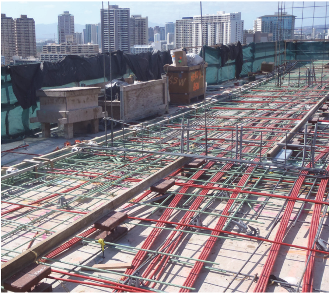
Fig. 2—PT slab under construction.
