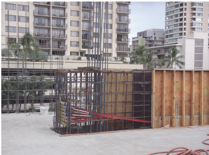
Fig. 7—PT upturn transfer girder.
