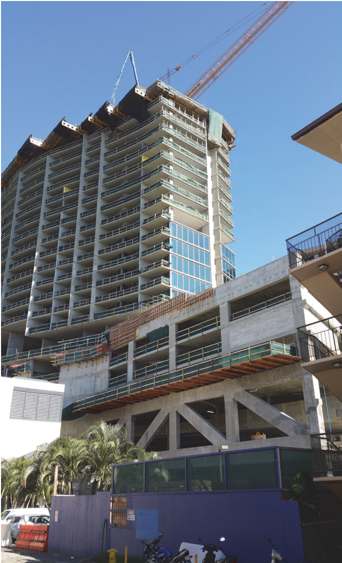
Fig. 10—PT concrete truss under construction.
