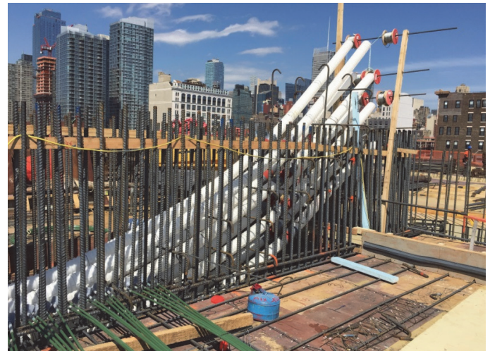
Fig. 8—PT wall under construction.
