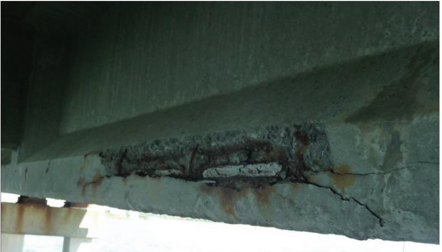
Fig. 1—Deteriorated beam exhibiting cracking, rust staining, spalling, and efflorescence.
