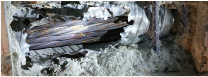
Fig. 7—Inspection opening in voided area.
