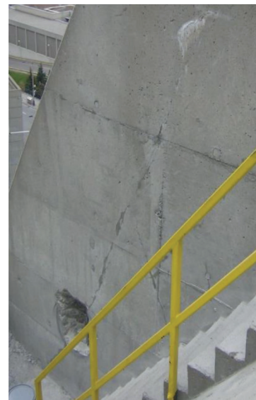
Fig. 2—Concrete showing efflorescence and cracking.
