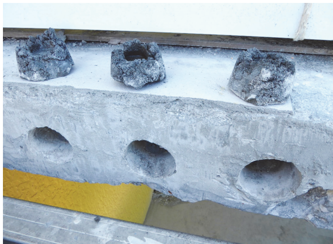
Fig. 20—Poor-quality grout with voids at stressing pockets.
