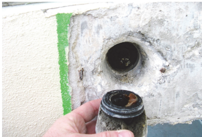
Fig. 21—Encapsulation cap not properly seated in anchor barrel bonded to grout plug.
