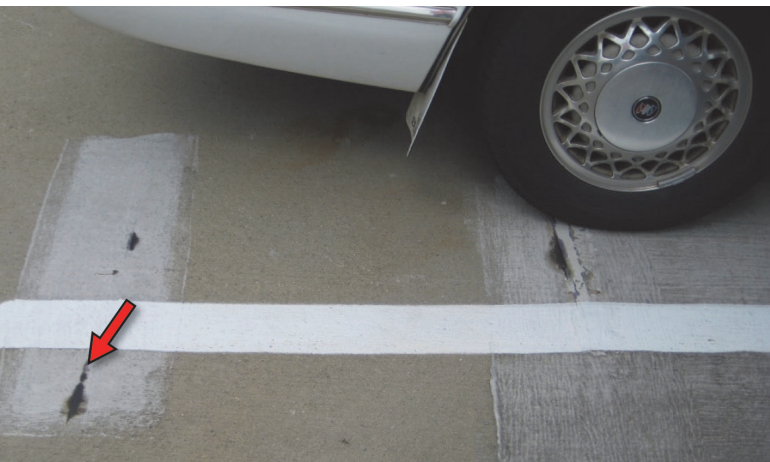
Fig. 11—Exposed PT sheathing and PT coating stains at top of slab.
