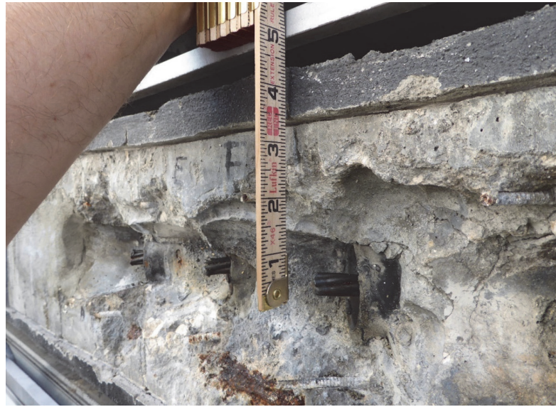
Fig. 18—Deficient strand tail length preventing proper seating of encapsulation caps.
