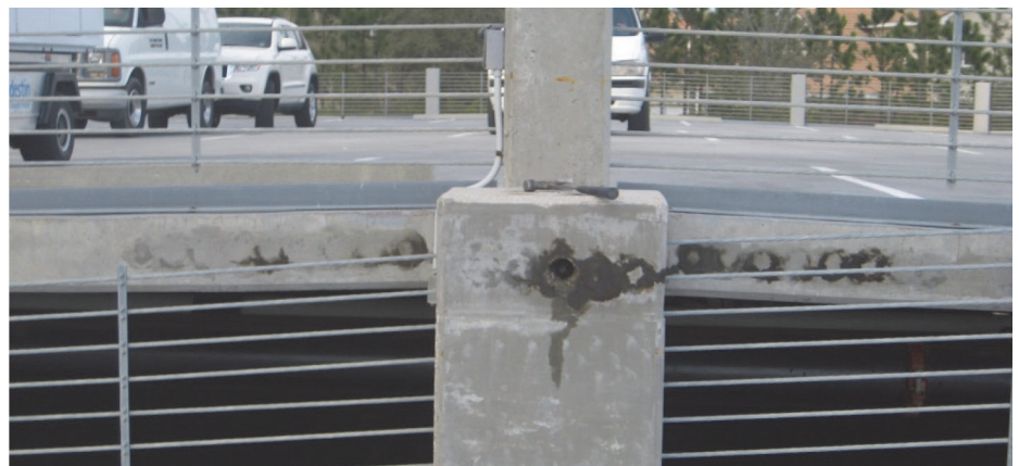
Fig. 9—Moisture emanating from grout pockets along elevated slab edge.
