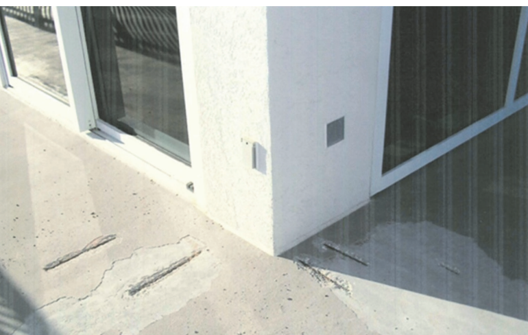
Fig. 1—Exposed reinforcing at balcony and corner column.
