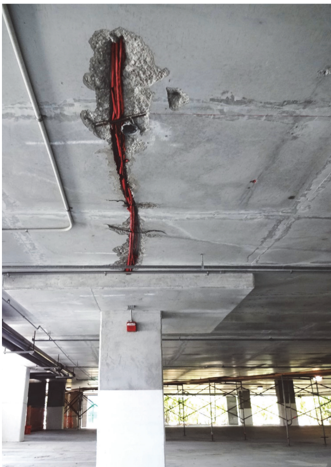
Fig. 6—Strand blowout with deficient horizontal and vertical PT strand alignment.
