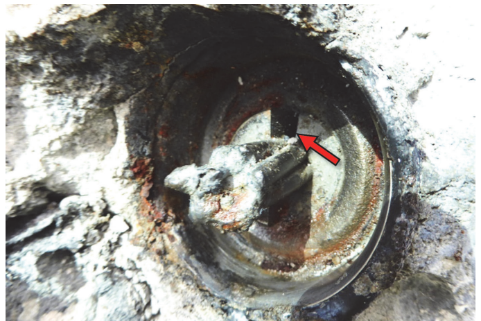
Fig. 19—Offset wedges at stressing anchor.
