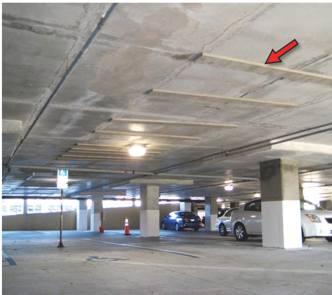
Fig. 5—Typical overhead patches aligned with uniform strands in parking structure.
