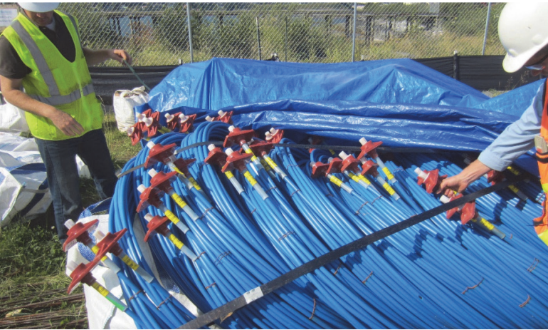
Fig. 16—Typical on-site storage with metal strapping.
