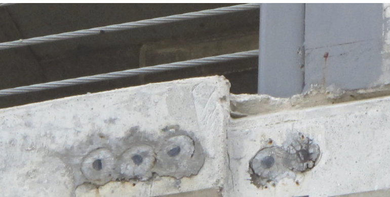
Fig. 12—Exposed encapsulation caps and voids in grout at stressing pocket.
