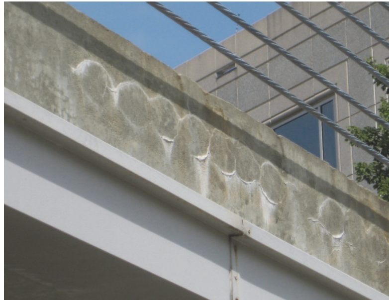
Fig. 13—Grout shrinkage at grout pockets with efflorescence emanating from grout pocket.
