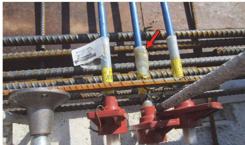
Fig. 14—Damaged PT sleeve prior to concrete placement.
