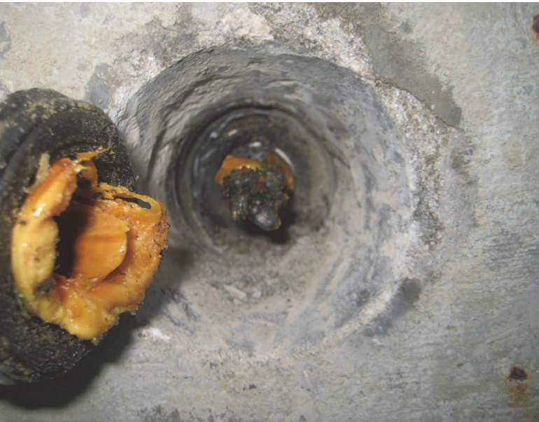
Fig. 10—Strand tail too long, encapsulation cap not seated, and emulsified PT coating.
