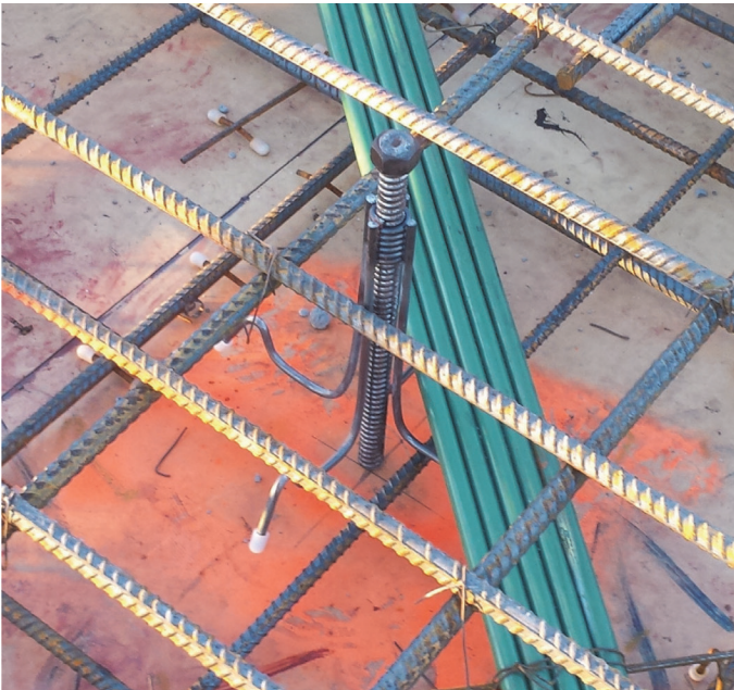
Fig. 11—Bolt used to mark relative location of scan data after tendons are covered in concrete.
