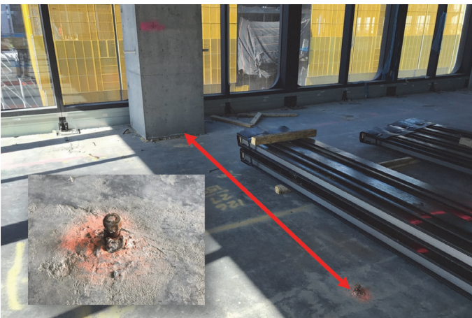
Fig. 12—Top of anchor bolt visible and available for measurement from columns.
