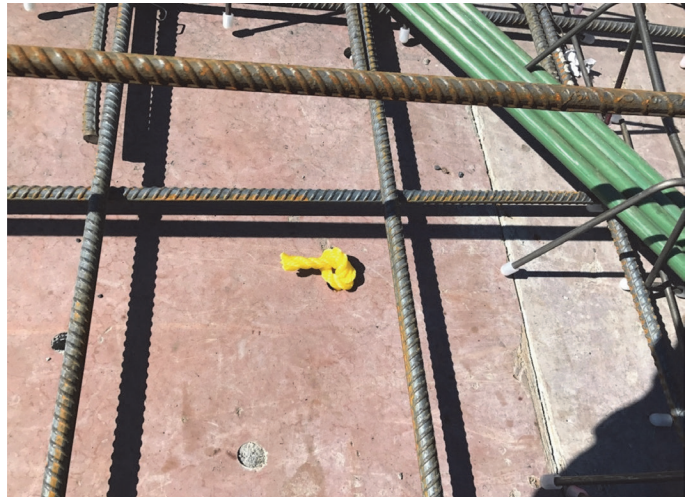
Fig. 4—Nylon rope used to mark outer boundary of tendon bands.
