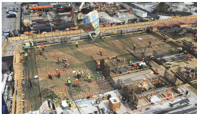
Fig. 3—Slab under construction showing layout of tendons.
