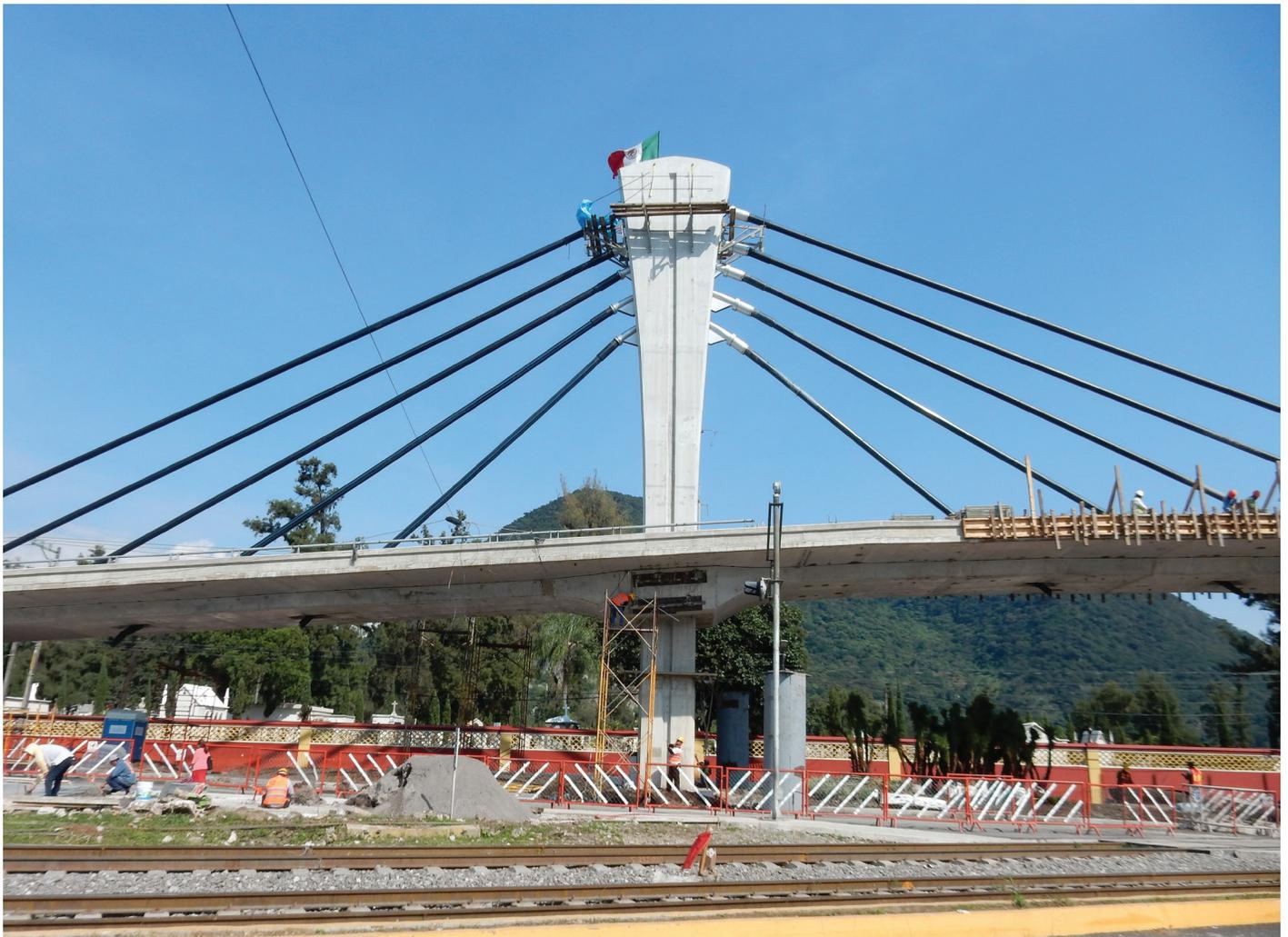
Fig. 4—Stay anchorage installation.
