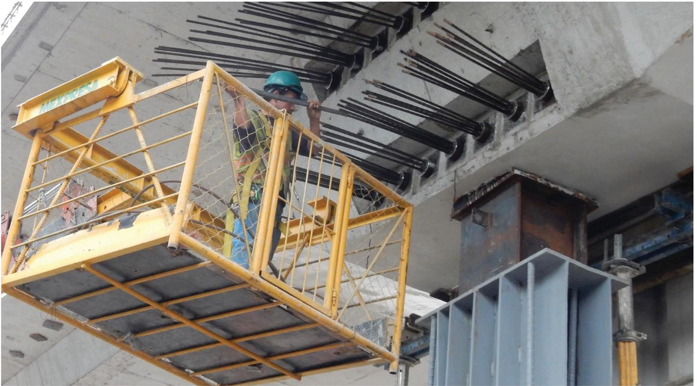
Fig. 8—Transverse deck post-tensioning.
