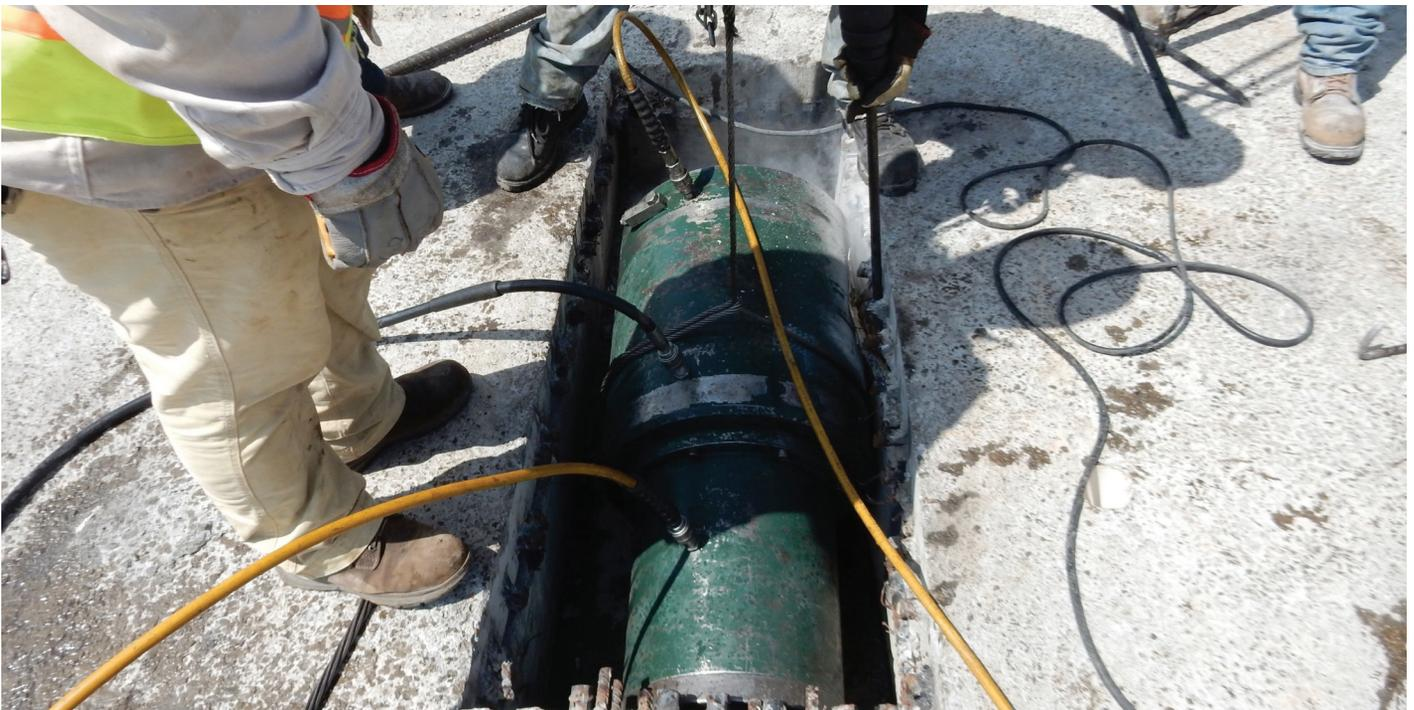
Fig. 7—Stressing of tendons from deck recesses.
