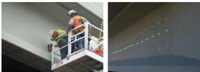
Fig. 2—(a) GPR to locate web tendons; and (b) tendon locations marked on girder web.
