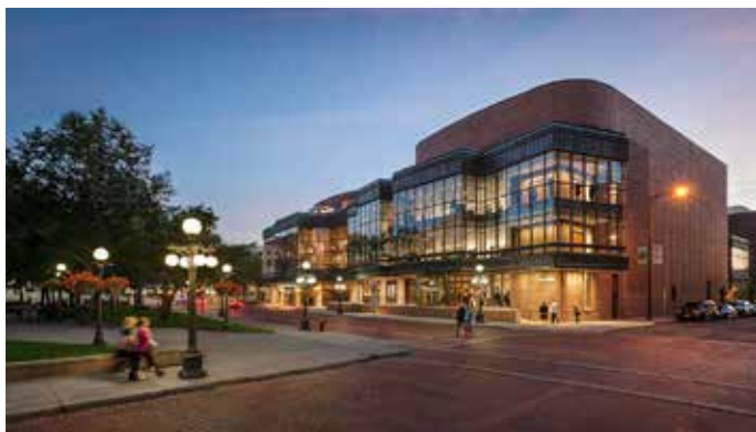
Fig. 4—Ordway Center for the Performing Arts Concert Hall Expansion.
