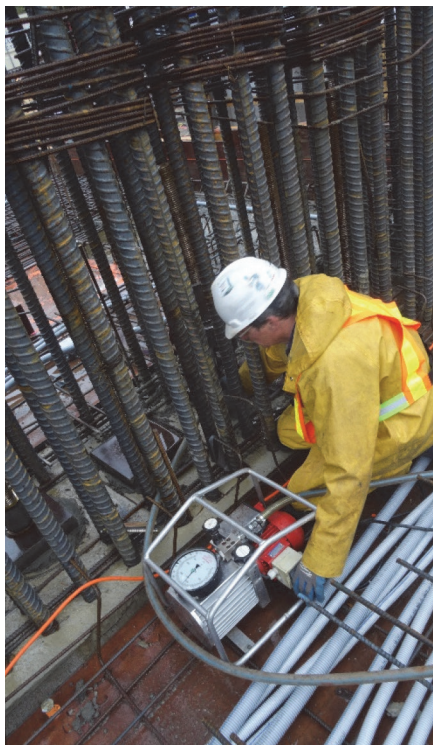
Fig. 5—Stressing of tendons at intermediate points.
