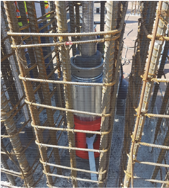
Fig. 4—Stressing of vertical threadbars.
