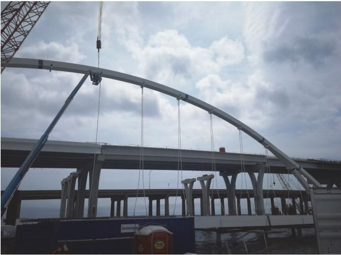
Fig. 5—Lifting of prefabricated hanger.
