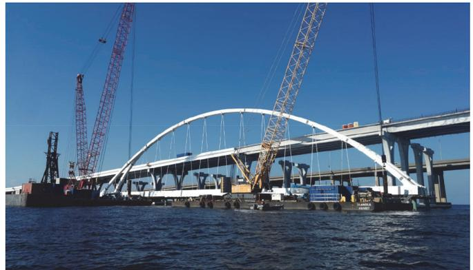
Fig. 7—View of bridge after completion of hangers prestressing.
