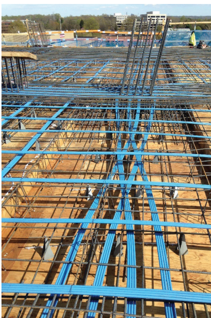
Fig. 6—PT distributed tendons crossed at midspan. Image Credit: DAVIS
