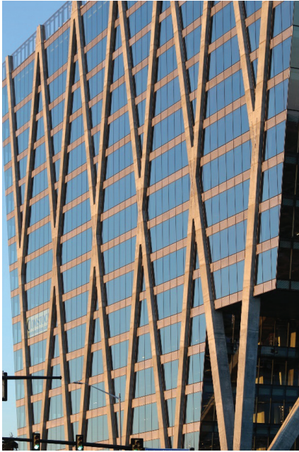
Fig. 5—Exoskeleton side view. Image Credit: Thornton Tomasetti
