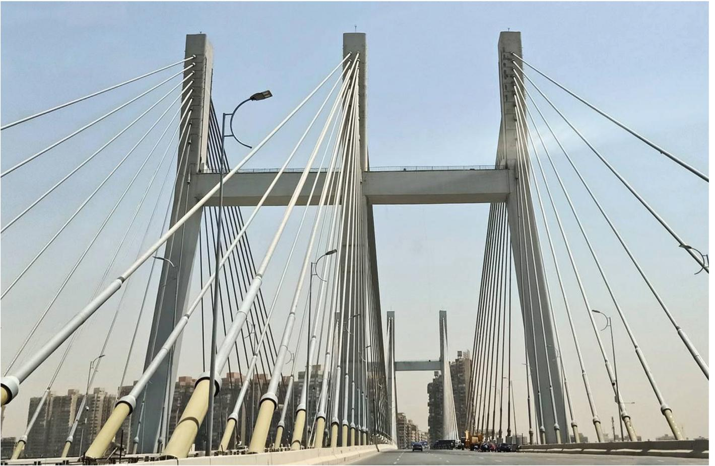
Fig. 2—Double H-shaped pylons.
