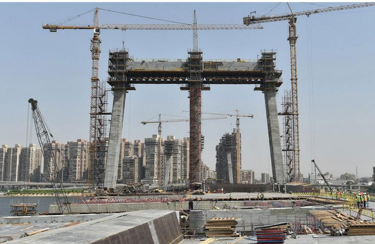
Fig. 7—Pylon construction using self-climbing formwork.
