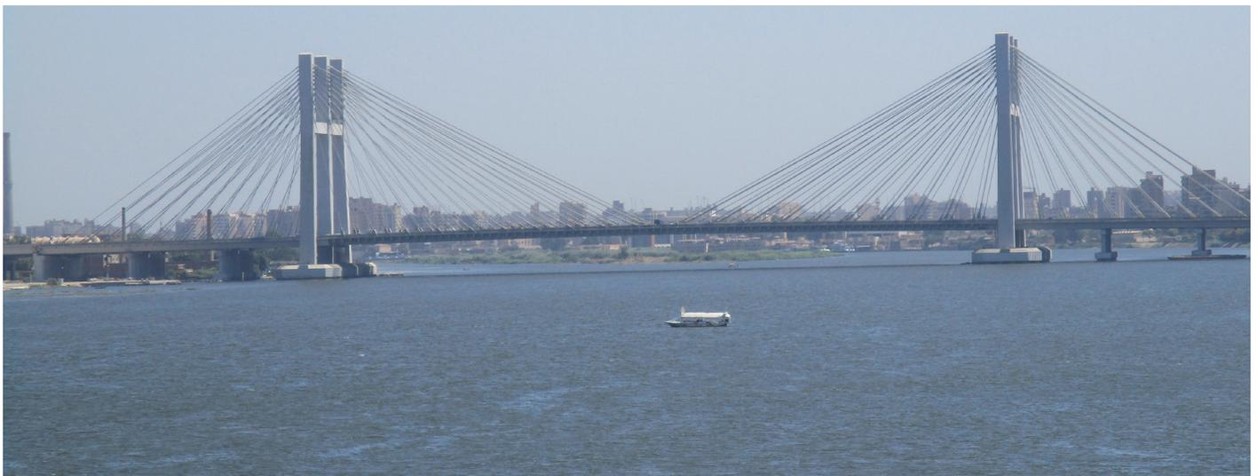
Fig. 4—Semi-fan arrangement of the cable stays.
