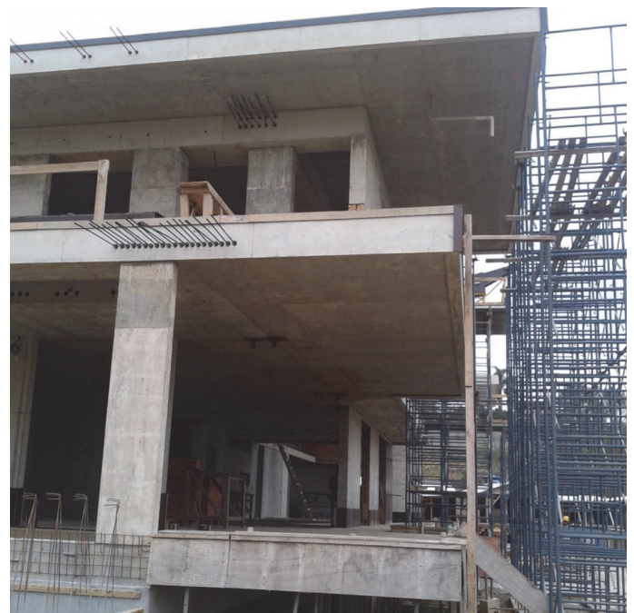
Fig. 5—Stayed column during construction.
