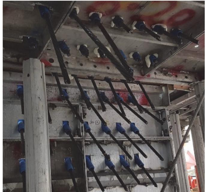
(a) Diagonal tendon anchorage, from beneath formwork
